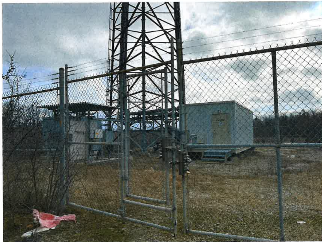
General view of electrical equipment adjacent to subject site to the North.
