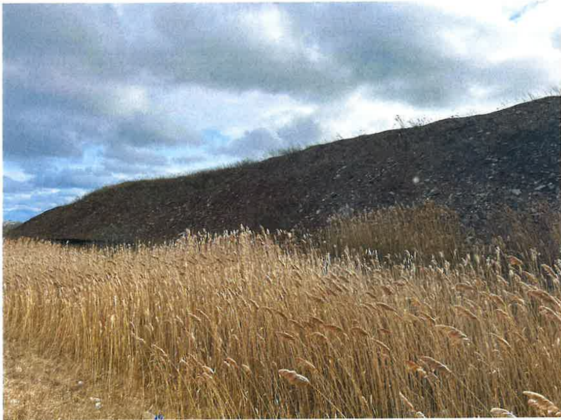
Closeup view of stockpile on eastern portion of subject site.
