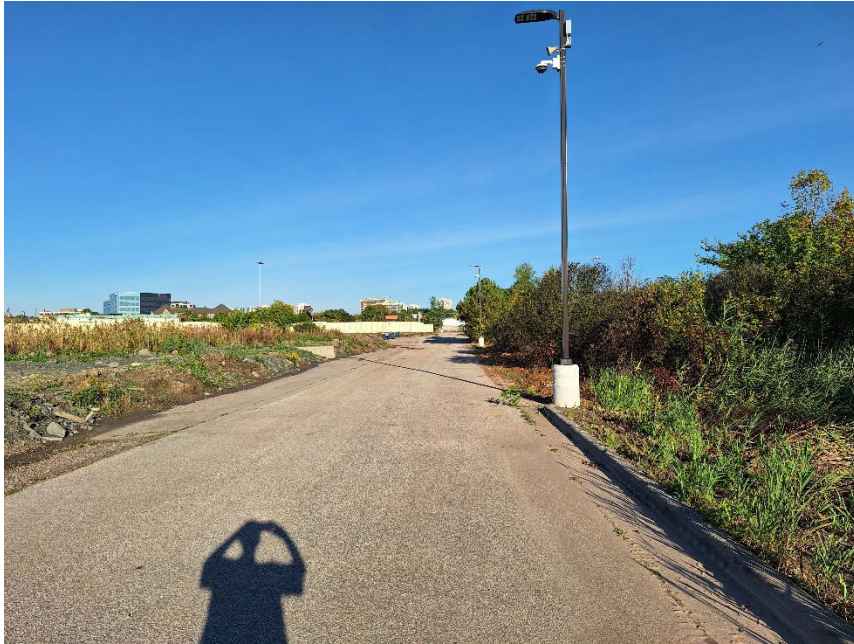
Image 17: View northwest along the road west of the drainage channel and berm.
