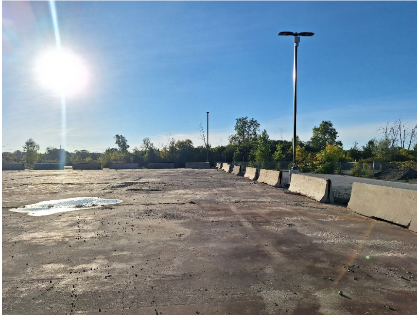
Image 3: View southeast across the factory floor slab.
