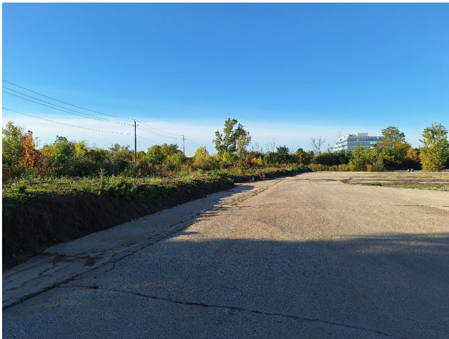
Image 6: View southwest along the edge of the pavements at the rear of the property where unauthorized piles of fill have been levelled out.
