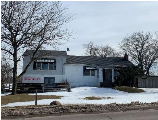
Picture 7: View of the south adjacent property, facing east.
