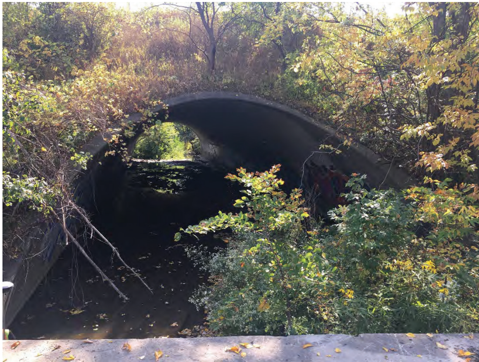
Photo 8 - Upstream Face of Royal Windsor Drive Culvert
