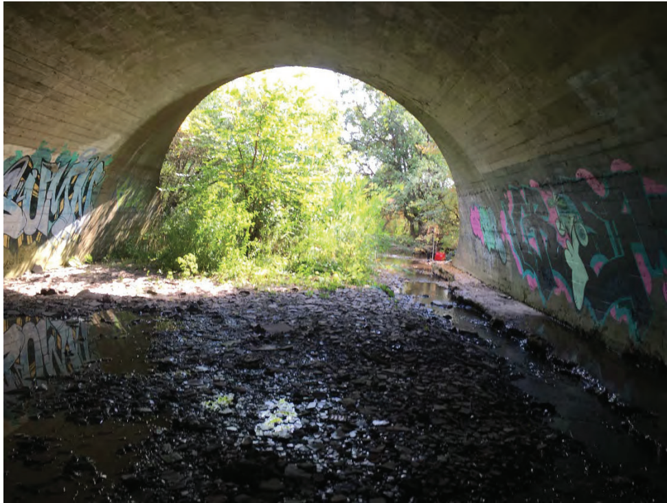
Photo 9 - Inside Barrel of Royal Windsor Drive Culvert
