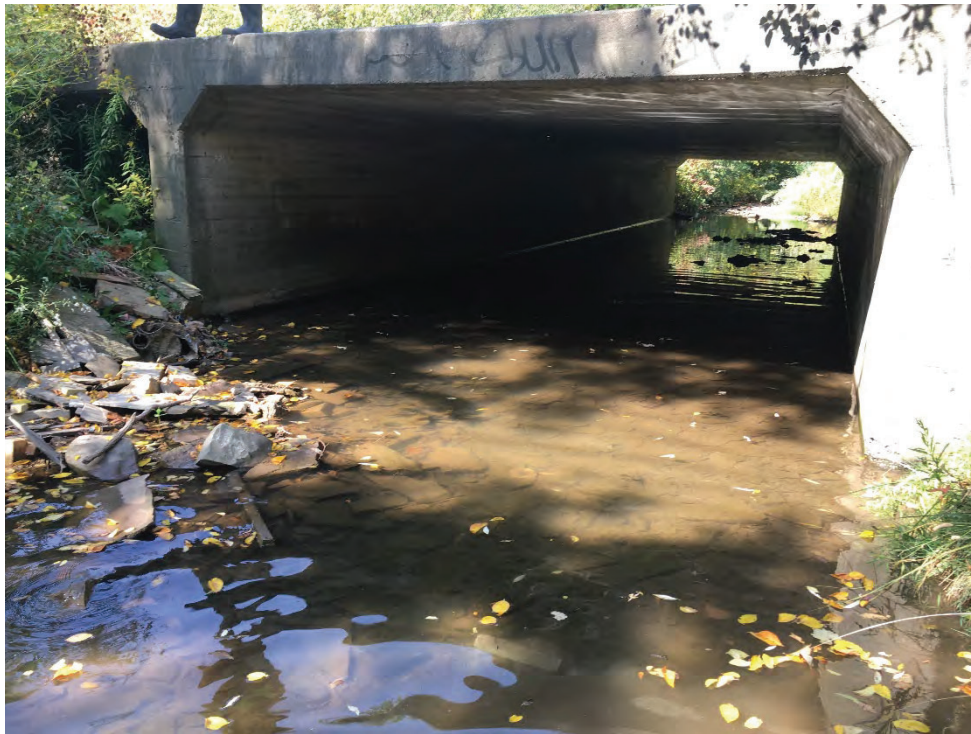
Photo 6 - Left Barrel of the Unnamed Service Road Culvert
