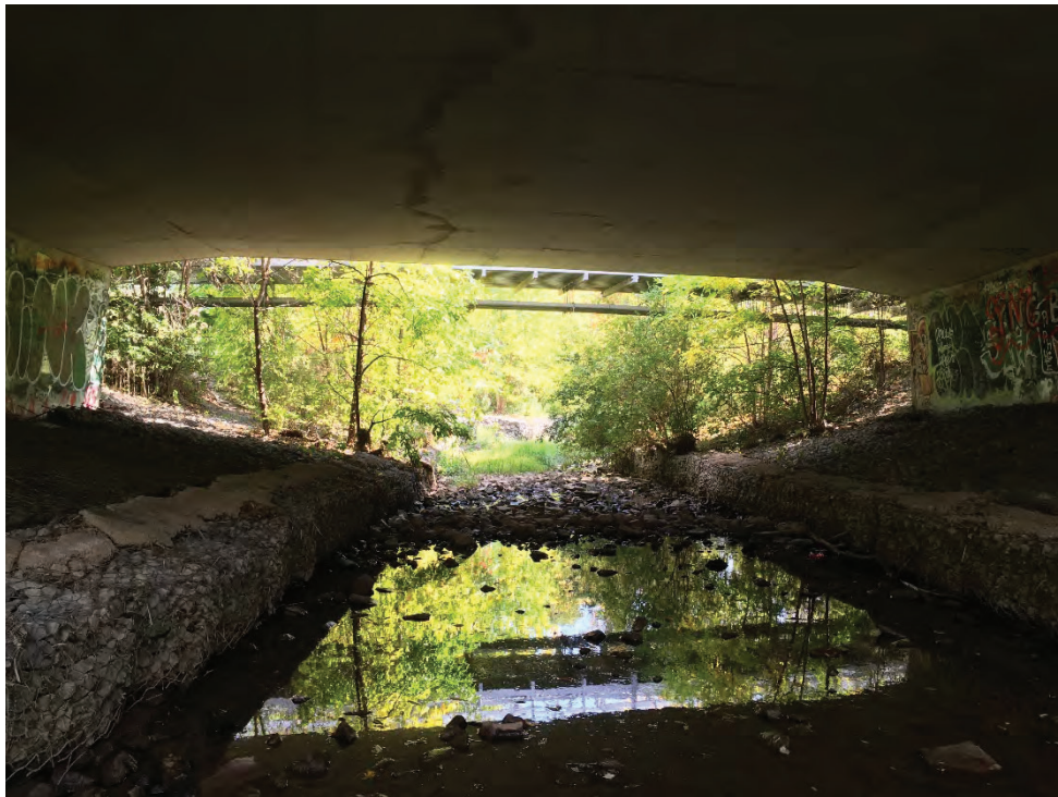
Photo 12 - Under Cornwall Road Bridge Looking Downstream
