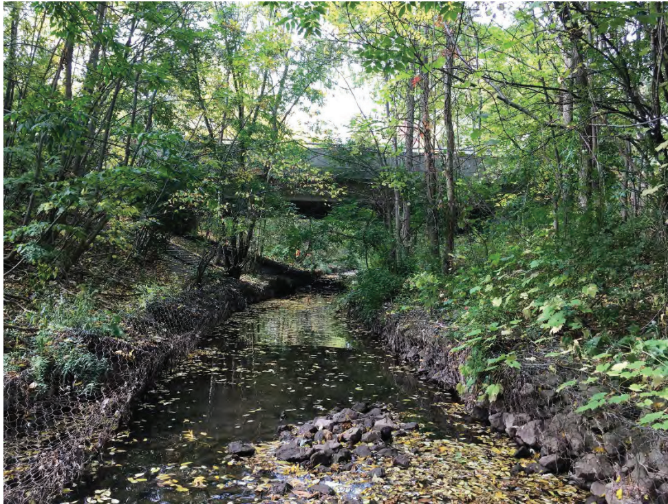
Photo 14 - Downstream Face of Constance Drive Bridge Looking Upstream
