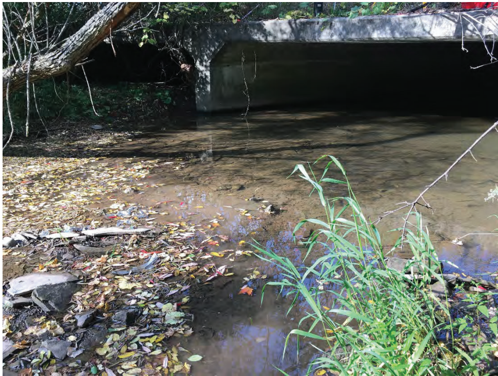
Photo 1 - Downstream Face of Private Road 2 Culvert Looking Upstream
