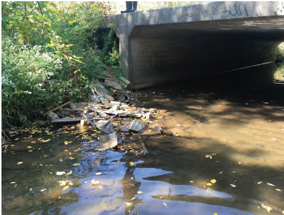
Photo 5 - Downstream Face of Unnamed Service Road Culvert Looking Upstream
