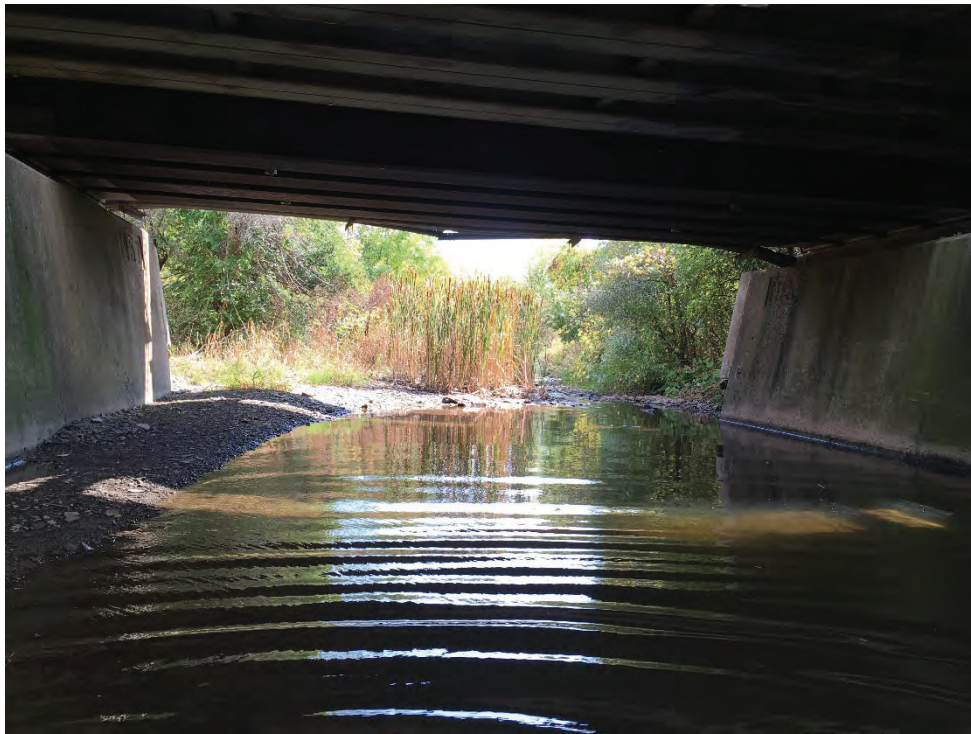
Photo 11 - Under the CN Rail Bridge Looking Downstream
