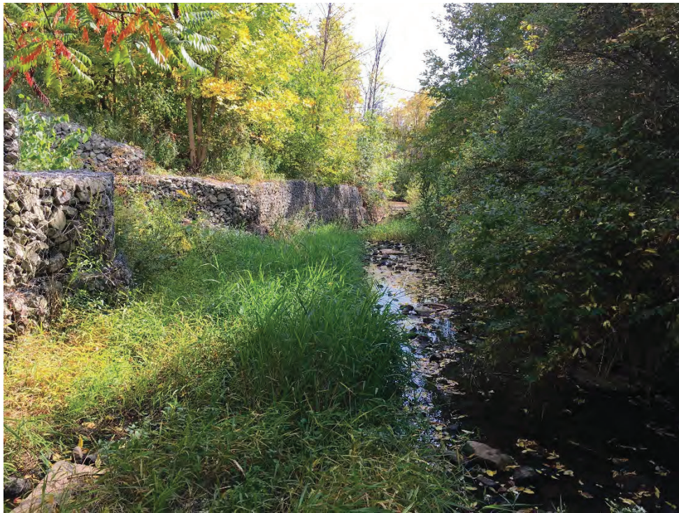
Photo 13 - Joshua's Creek Downstream of the Cornwall Road Bridge
