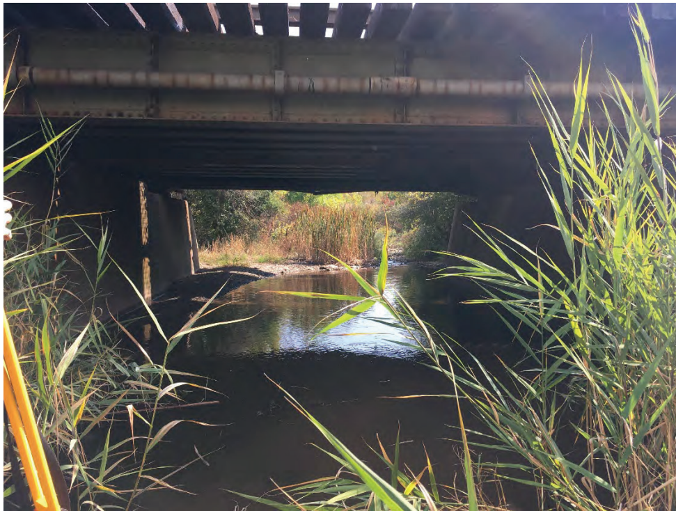
Photo 10 - Upstream Face of CN Rail Bridge
