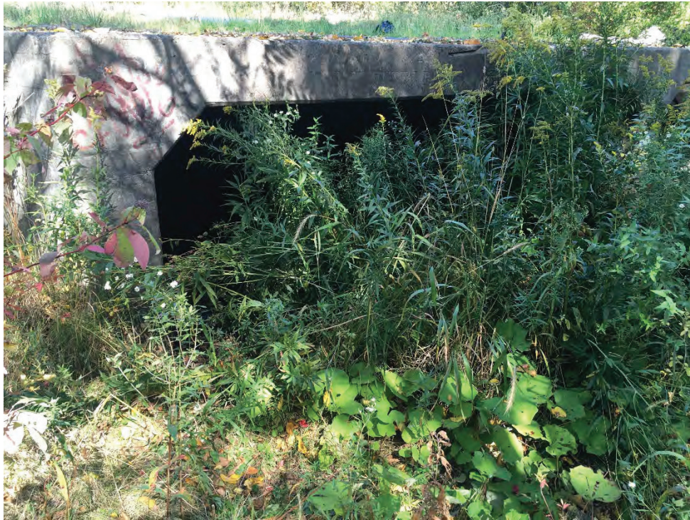
Photo 7 - Right Barrel of the Unnamed Service Road Culvert
