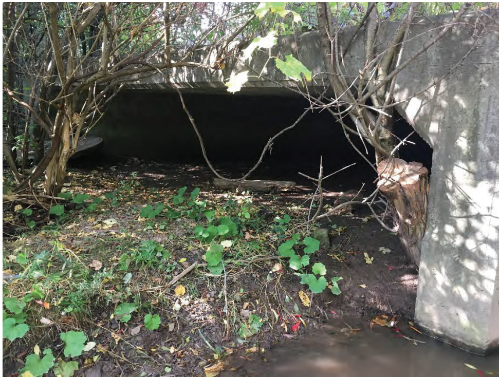
Photo 3 - Right Barrel of the Private Road 2 Culvert
