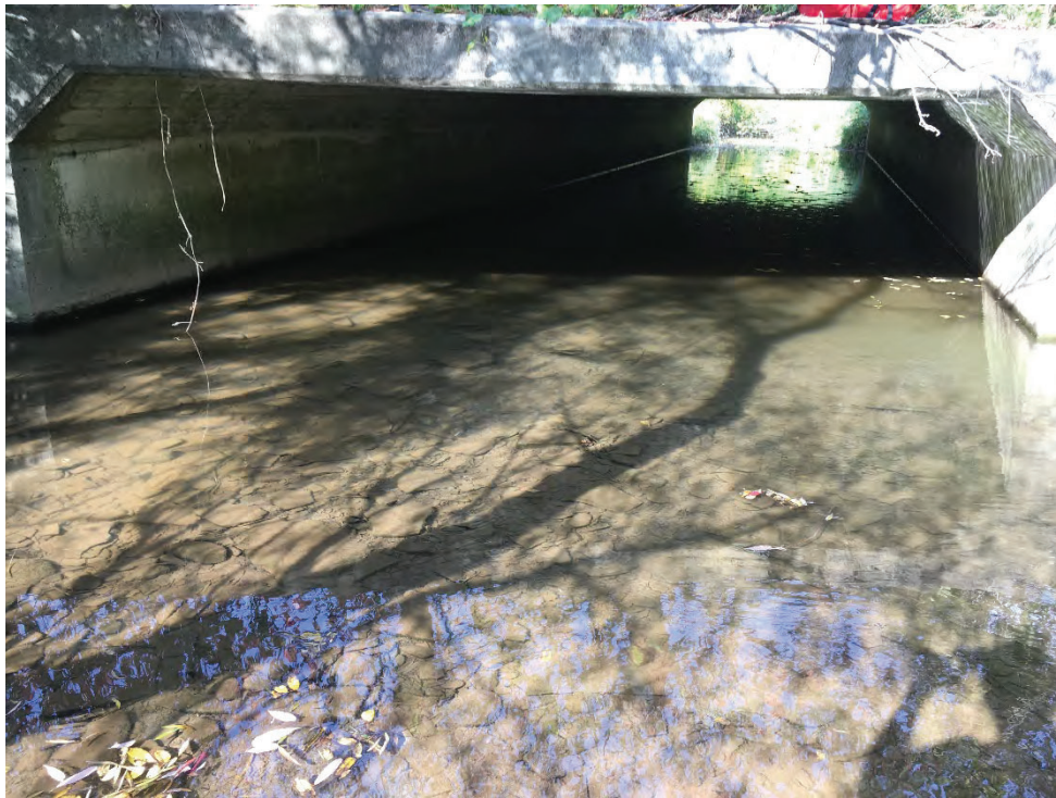
Photo 2 - Left* Barrel of the Private Road 2 Culvert
