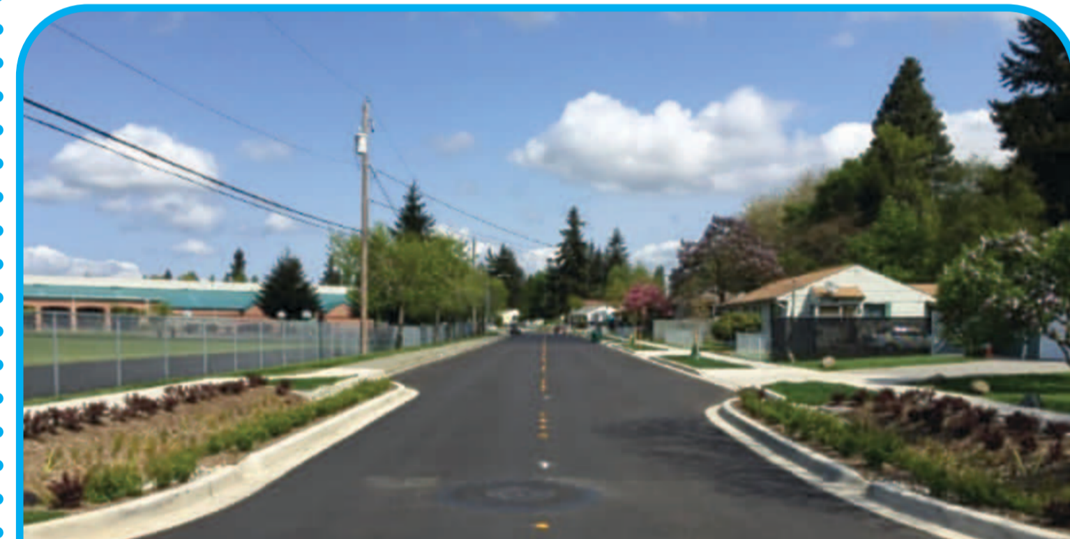
Rain gardens and bioretention curb extensions
