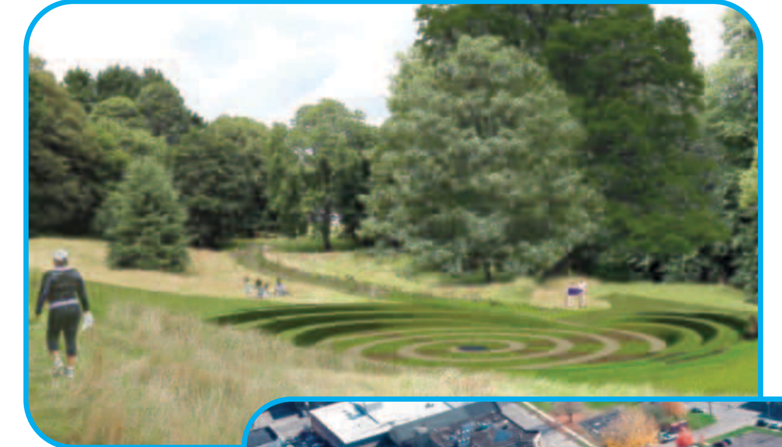
Dry pond – above-ground temporary water storage
