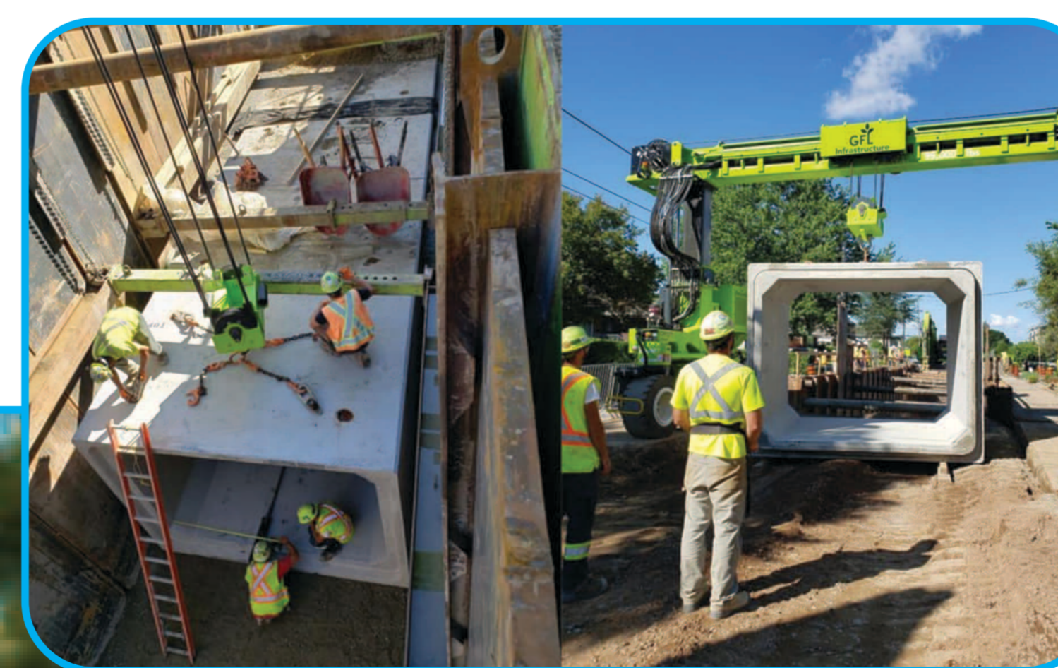
Storm sewer upsizing and superpipe storage
