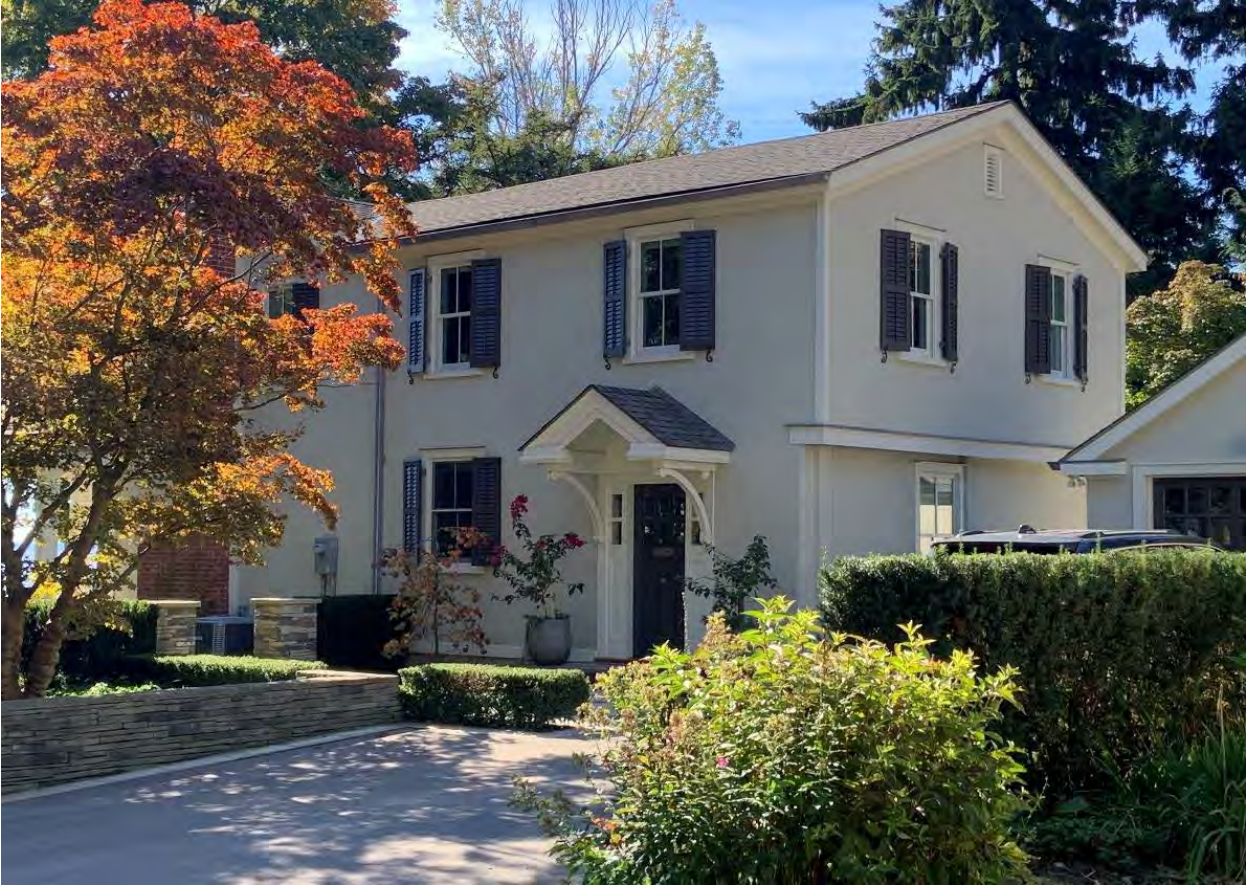
22 Reynolds Street – Example of Stucco Cladding
