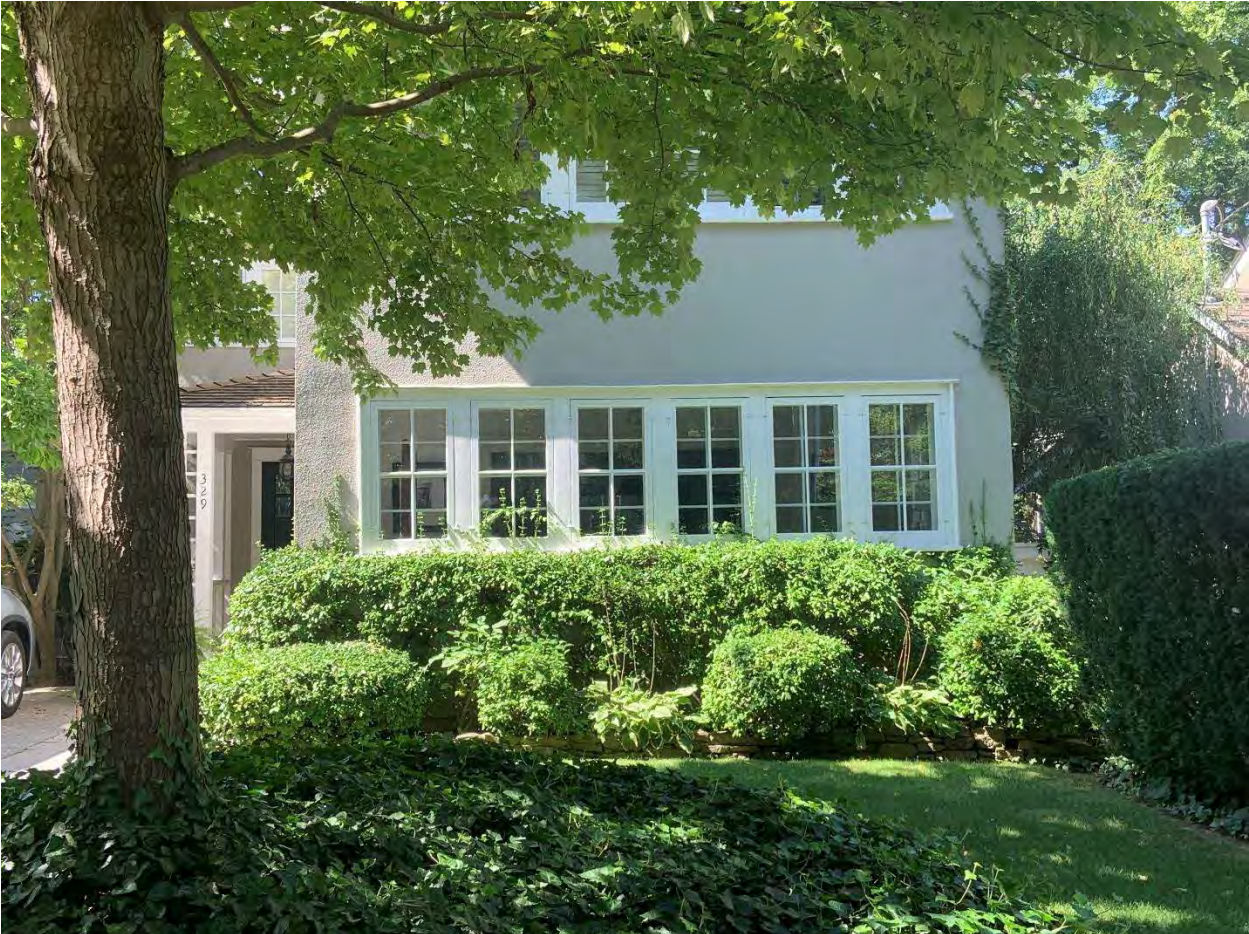
329 William Street - Wood Windows with storms
