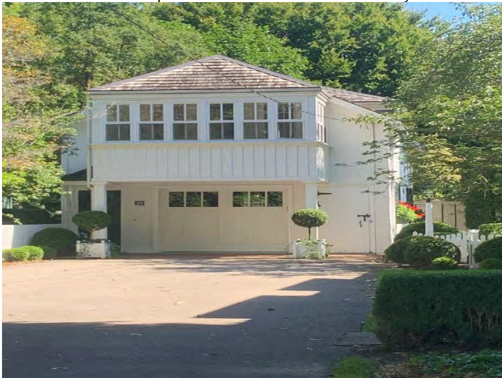
53 Navy Street – Coach House set back and facing William Street away from main residence
