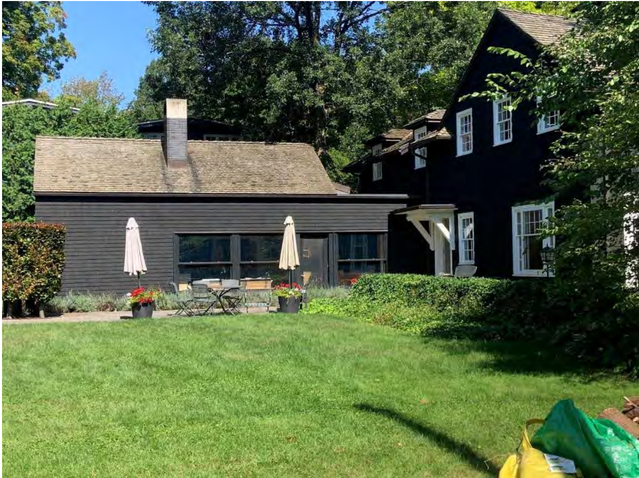
King Street – small addition to rear and visible from side yard facing George Street. One storey “connection” to original creates impression of outbuilding; complementary gable shake roof and use of colour; distinction in cladding through use of horizontal wood and in window form
