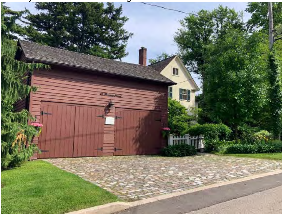
29 Thomas Street – Detached Garage (restored barn)
