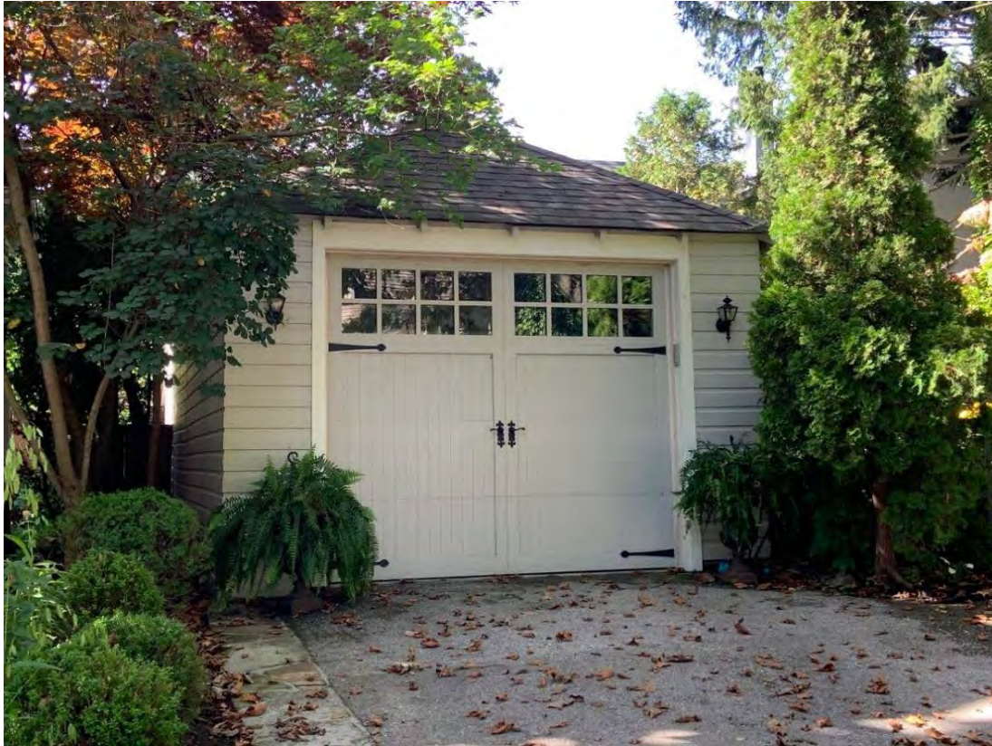
32 Thomas Street – Detached Garage
