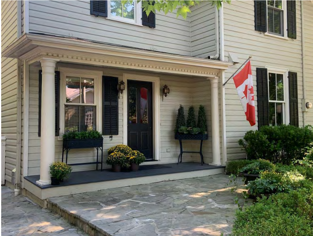
53 Dunn Street – Example of Horizontal Wood Cladding
