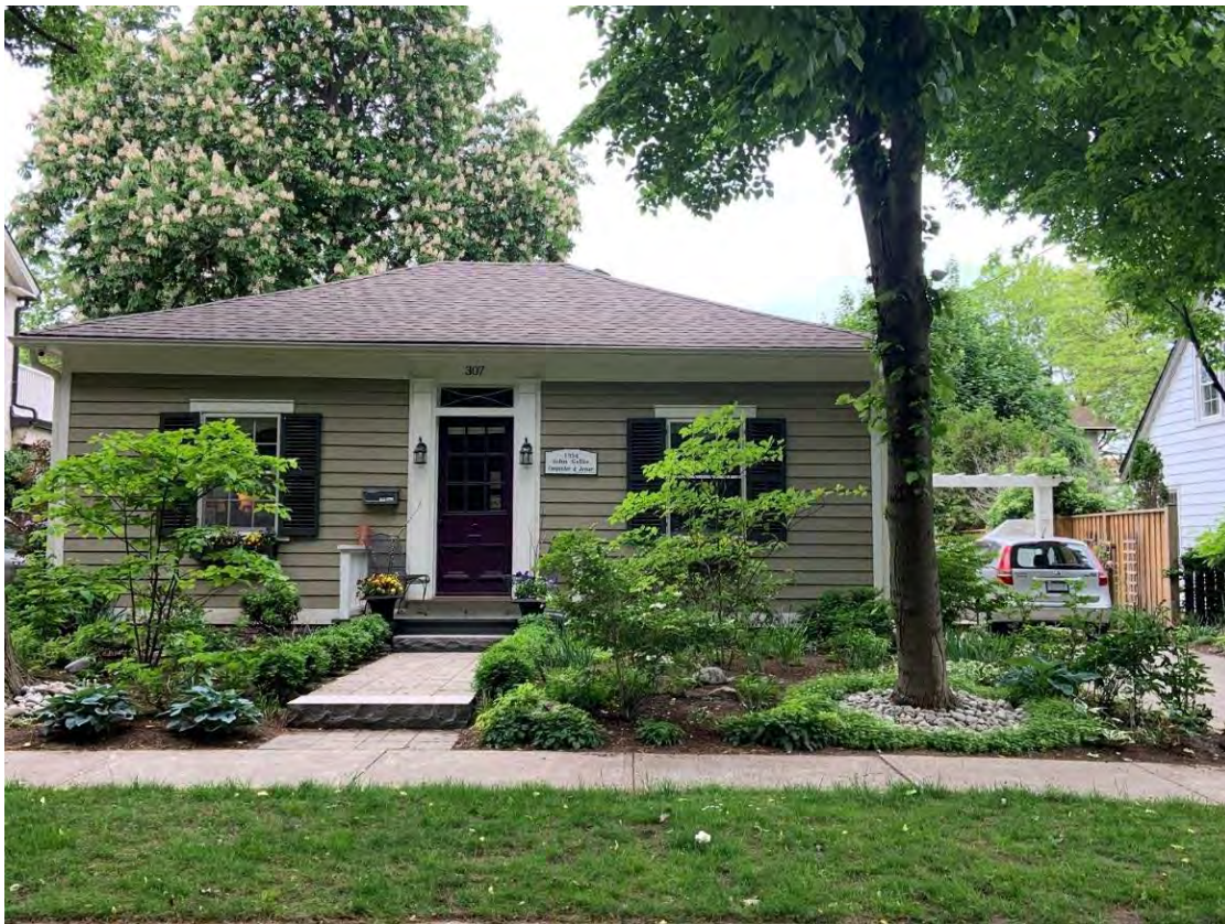
307 William Street – Asphalt Hip Roof with Horizontal Wood Cladding
