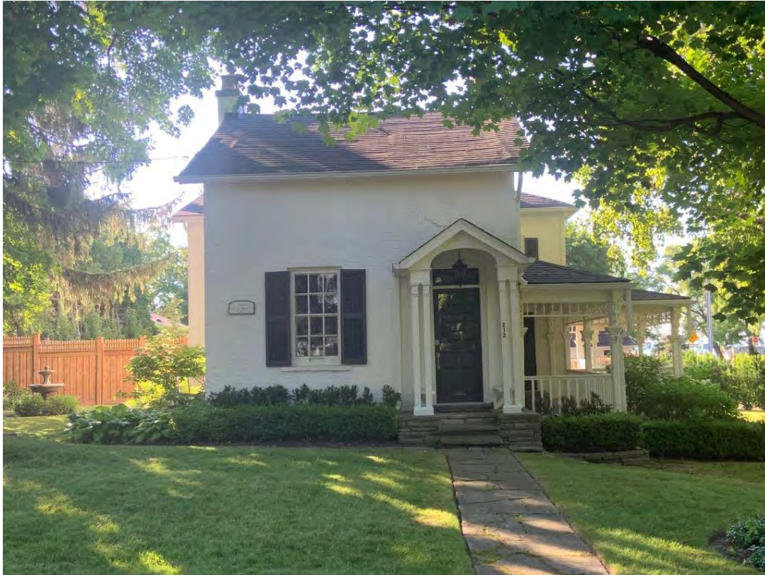
212 King Street – Main Entrance Wood Door facing street
