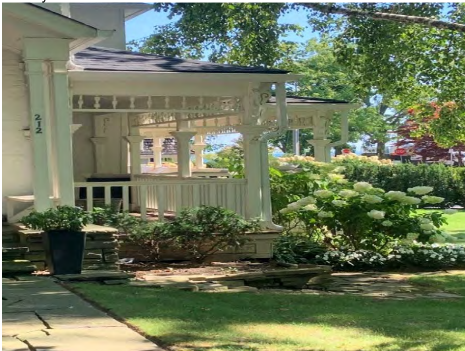
212 King Street – Covered Open Porch
