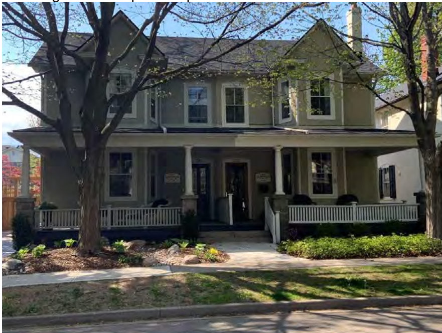
295 & 297 William Street – Open Front Porch
