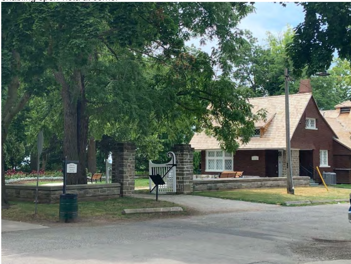
Navy Street Erchless Estate – low stone wall with stone pillars and wooden gate
