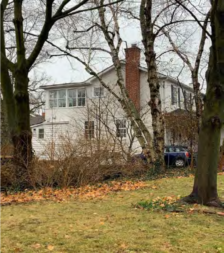
188 William Street –addition to rear and visible from William Street. Height of addition is lower than original, combination of consistent stucco cladding and complementary horizontal wood cladding; wood windows in complementary style
