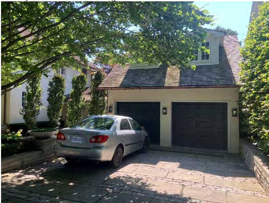
66 Dunn Street – Attached 1 ½ Storey Garage with appearance of detachment through single storey connection to main residence
