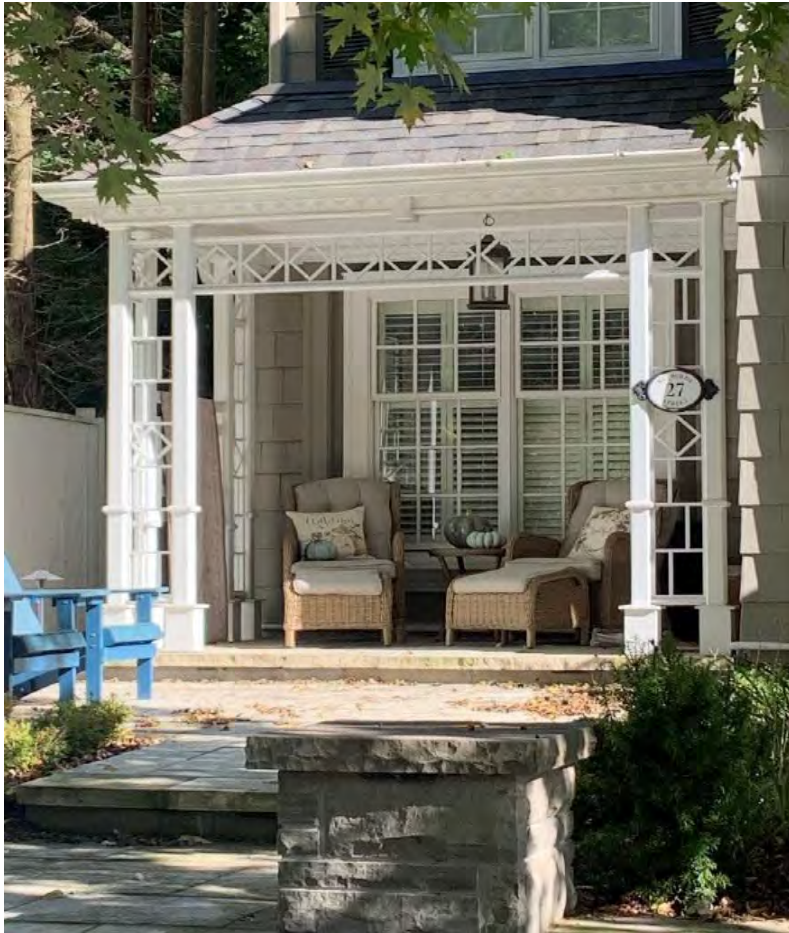
27 Reynolds – Covered Porch
