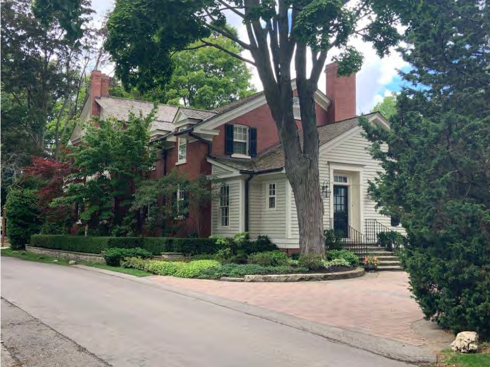
19 Navy Street – addition to rear and visible from side street; height of addition steps down; consistency in roof form and style of windows/doors and trim; complementary use of materials including brick and horizontal wood cladding
