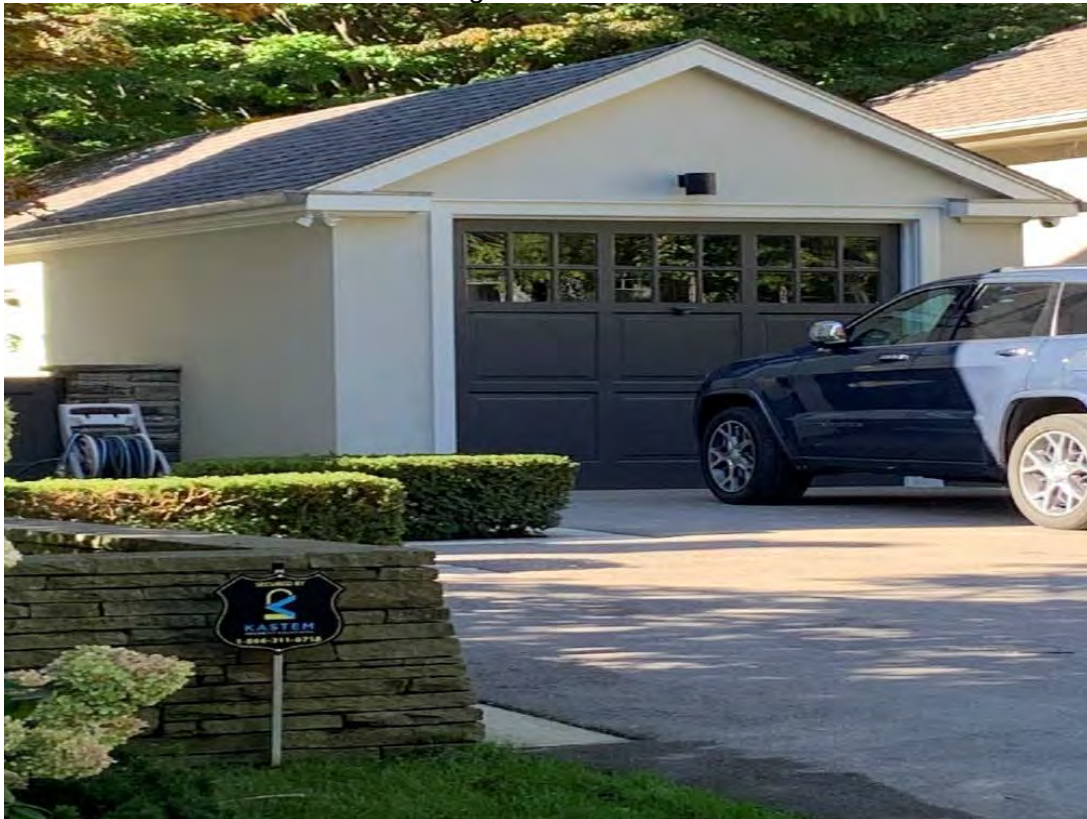
22 Reynolds Street – Detached Garage
