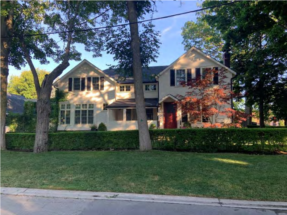
273 William Street – addition to west; height of addition matches; consistency in roof form and style of windows/doors and trim; complementary use of materials
