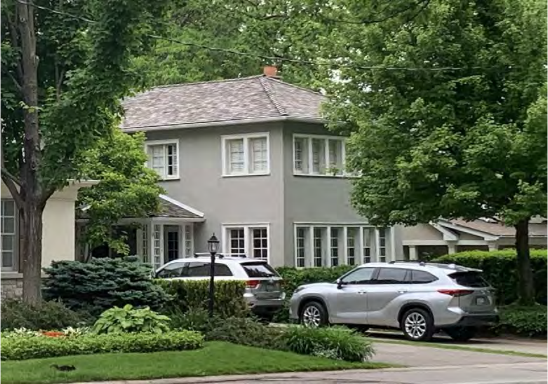
329 William Street – Cedar Shake Hip Roof with Stucco Cladding
