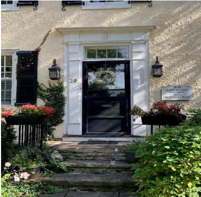
29 Navy Street – Main Entrance Wood Door with Surround facing street
