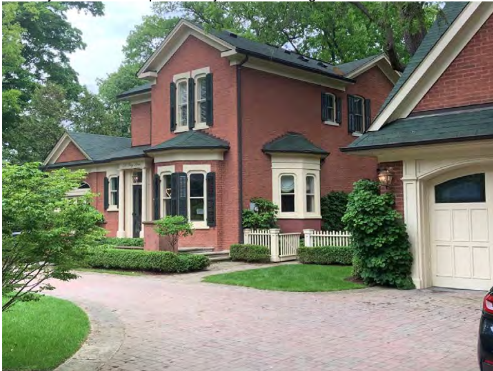
350 King Street – Example of Late 1800s Brick Cladding
