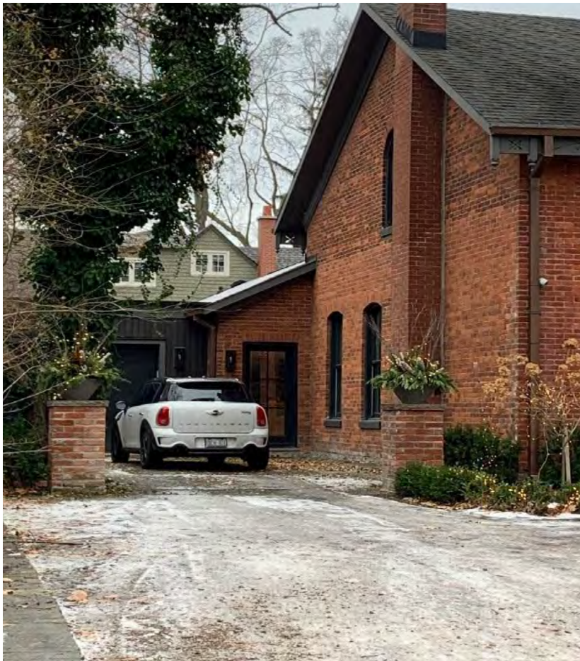
Trafalgar Road – Attached single car garage with shed appearance setback to rear of property
