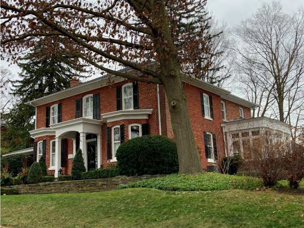
226 William Street – low lying lakestone wall across front of house with soft landscaping and open vistas to westerly side yard
