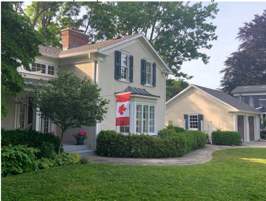
65 Navy Street – Asphalt Gable Roof on House and Garage with Stucco Cladding
