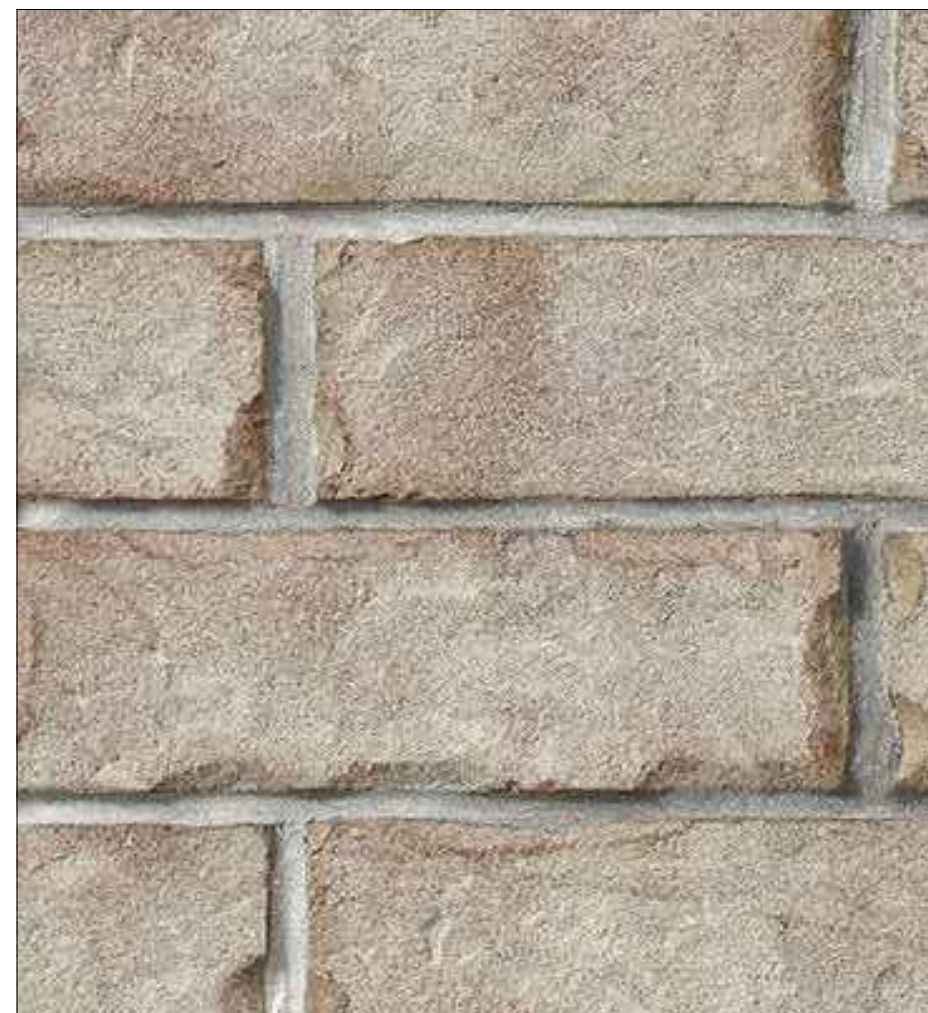
BRICK - BR04 UPPER PODIUM LEVEL BRICK MERIDIAN STRATHROY
