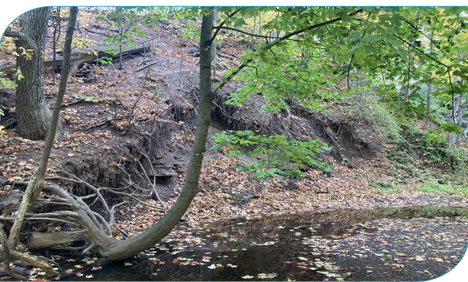
Site: E7, E9 Score: 56, 53 Issue: Toe erosion of valley slope (unprotected) Risk: Private property (parking lot) Length: 10 – 20 m
