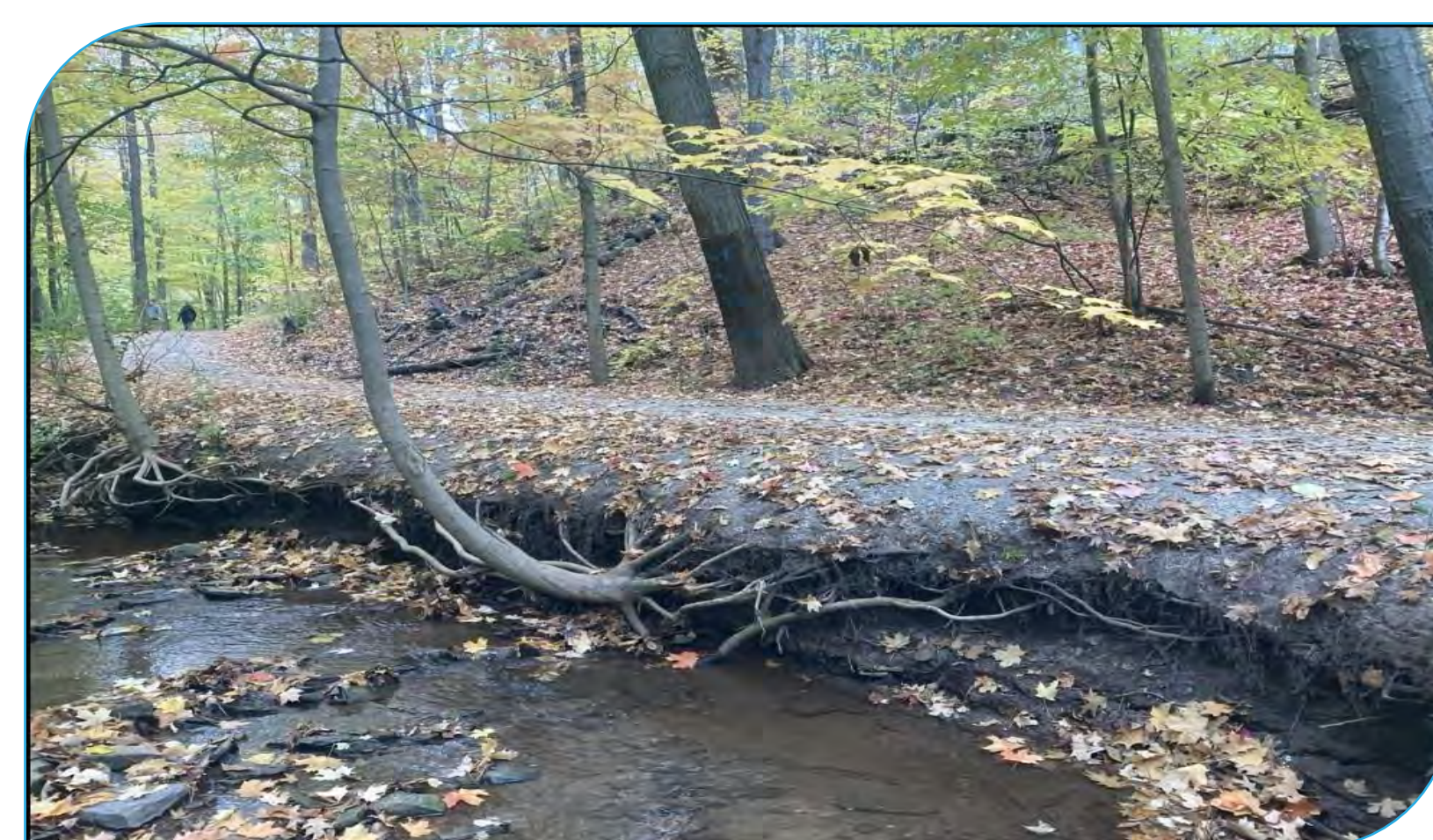
Site: E1, E2, E3, E8, E12, E13 (not included in EA) Score: 35, 26, 34, 38, 42, 43 Issue: Bank erosion in proximity to pedestrian trail system; not valley contacts. Risk: Mainly pedestrian trail system, pedestrian bridge (E13), secondary infrastructure (stormwater outfall - E12) Length: varies
