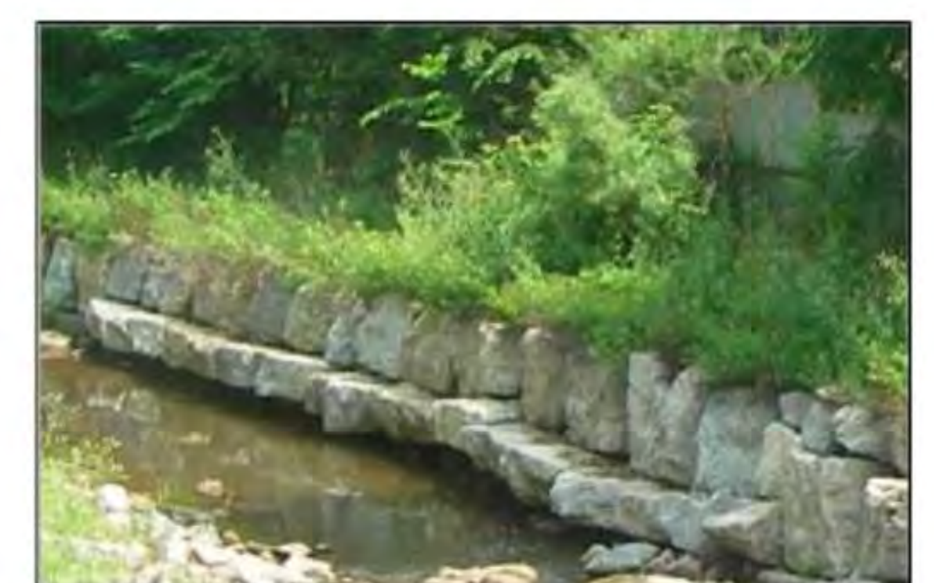
Armour Stone Wall with Brush Layer Concept
