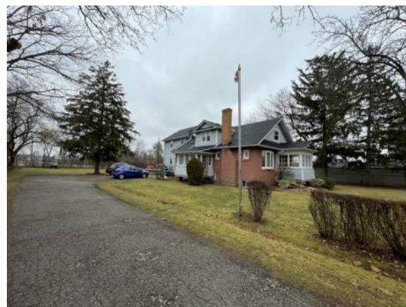
Photo 6: View of the north side of the Site building from the north-central portion of the Site. Photograph taken facing east.
