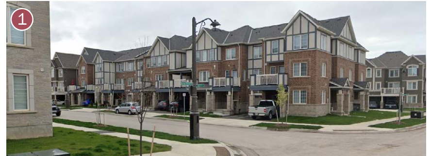
Existing recently constructed back-to-back townhouse units south east of Block 154
