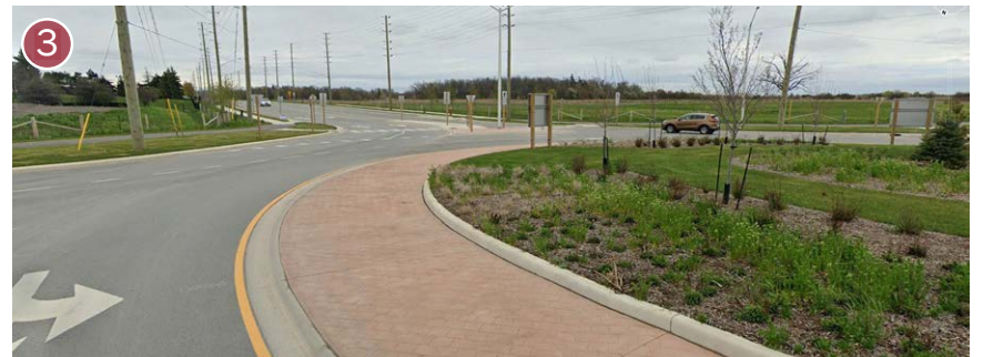
Newly constructed roundabout at William Halton Parkway and Sixth Line
