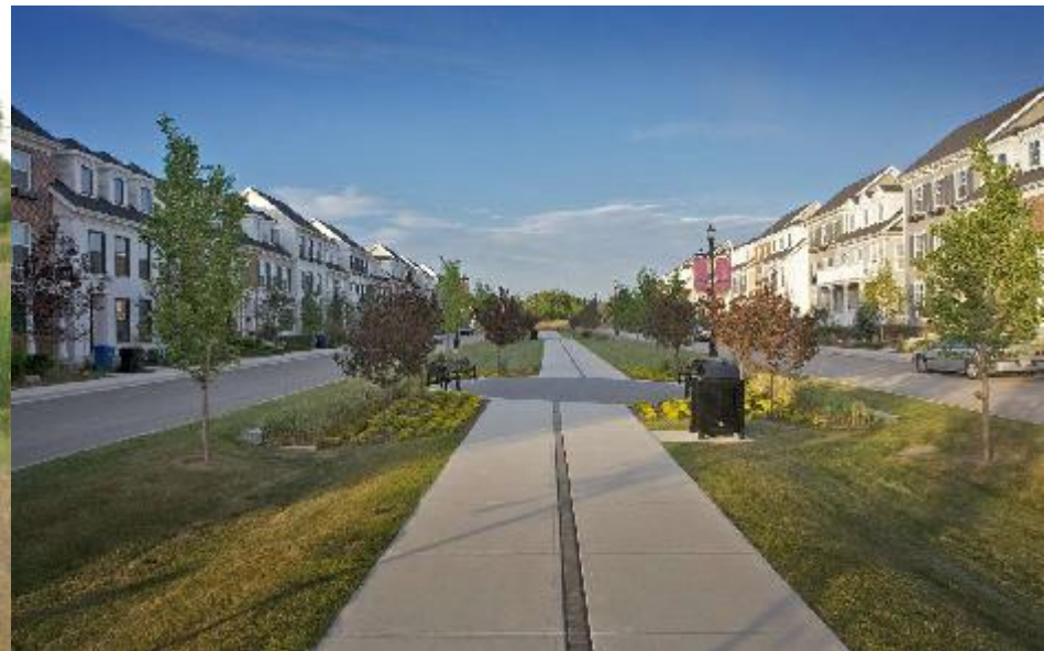
Bioretention System (Infiltrates drainage from roadways)
