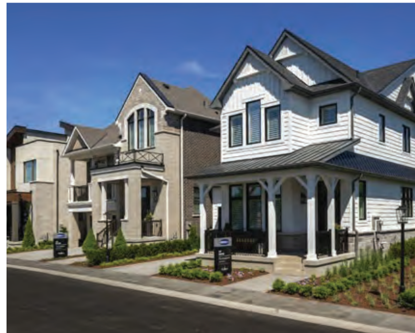
Figure 6.3.2b - Single detached dwellings with 2-storey massing should offer a variety of designs that include prominent porch entries as well as articulated facade treatments
