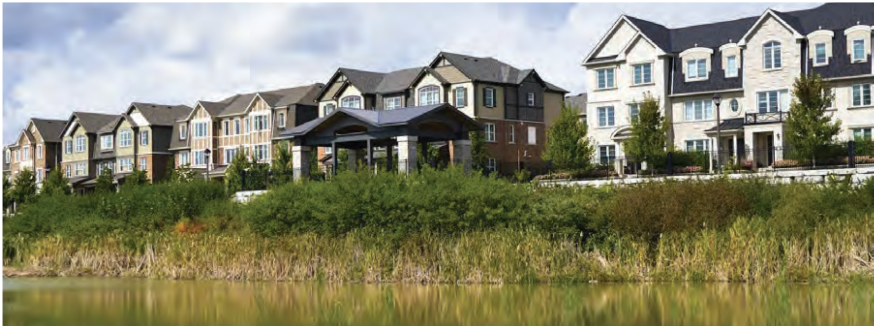
Figure 6.3.3 - Image example of 2-storey with prominent covered porch.
