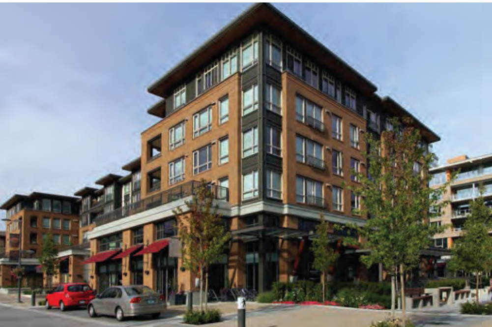
Figure 6.2.1a - Image example of a mixed use building with commercial ground floor units that establish an active urban character.
