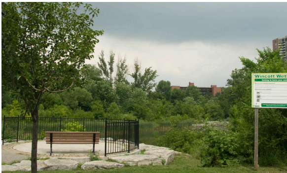
Public feature at storm water management facility
