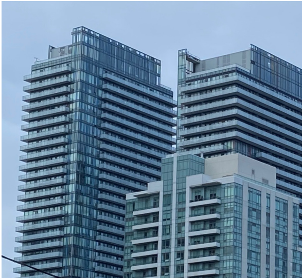
Mechanical rooms screened through structures that complement the overall building design
