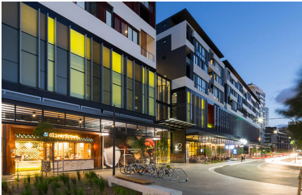
Courtyards and breaks in the building's massing height provide relief for long elevations
