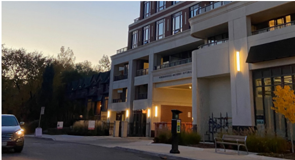
Consolidated access to underground parking and internalized servicing/loading areas, provided from a secondary street
