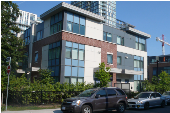
Wrap-around windows, side main entrances and articulated designs are used to address corner conditions
