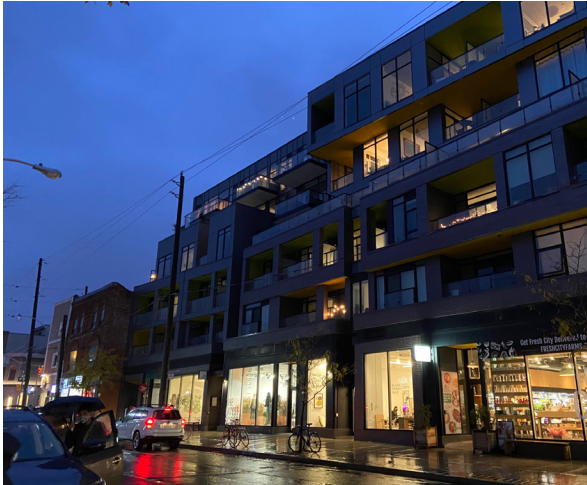
Strategic use of glazing differentiates uses on the same elevation
