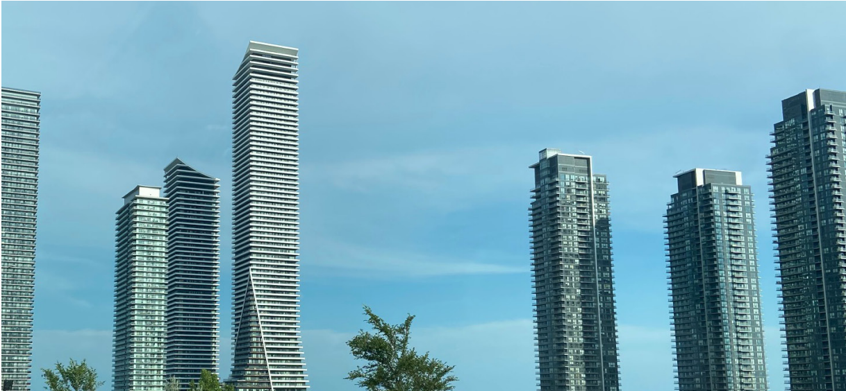
Staggered towers of various heights and small floorplates result in an animated skyline and maximized sky views.
