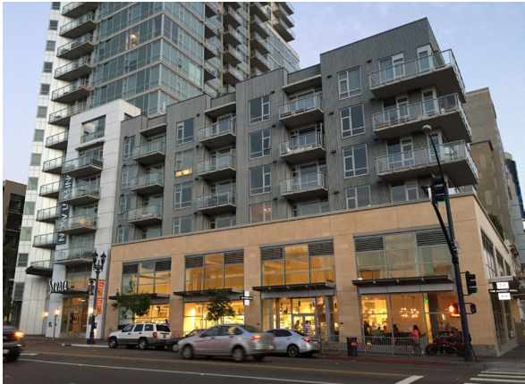
Taller ground floor emphasizes the presence of habitable spaces along the streetscape and provides for flexibility in at-grade uses
