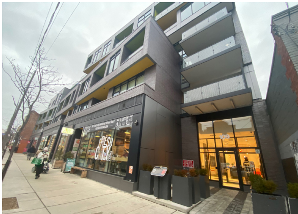
Different uses on the same elevation are accentuated through different setbacks, stepbacks and architectural treatments
