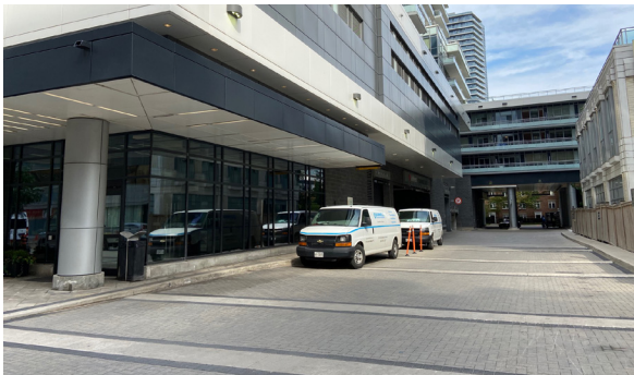
Servicing/loading areas and access to underground parking located to the side of the building, away from the public realm
