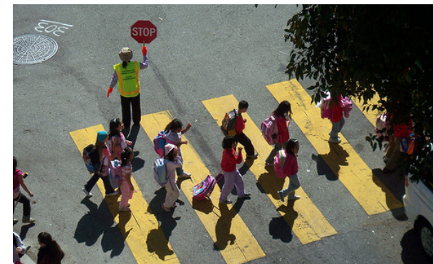
Marked pedestrian crosswalks
