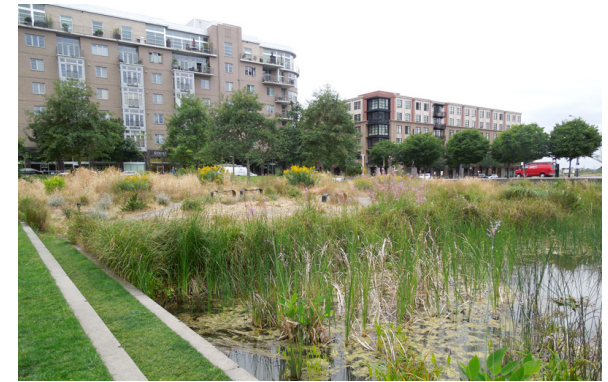
Naturalized SWM Facility
