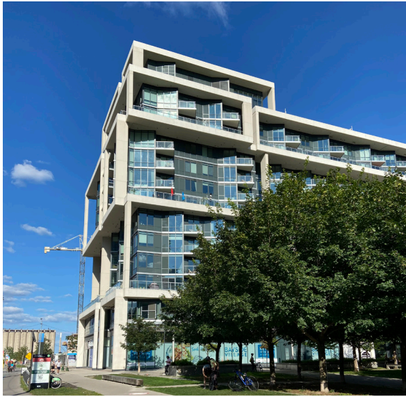
Enhanced corner treatment, with taller component at the corner, equally addresses both elevations with highly articulated design and complementary materials
