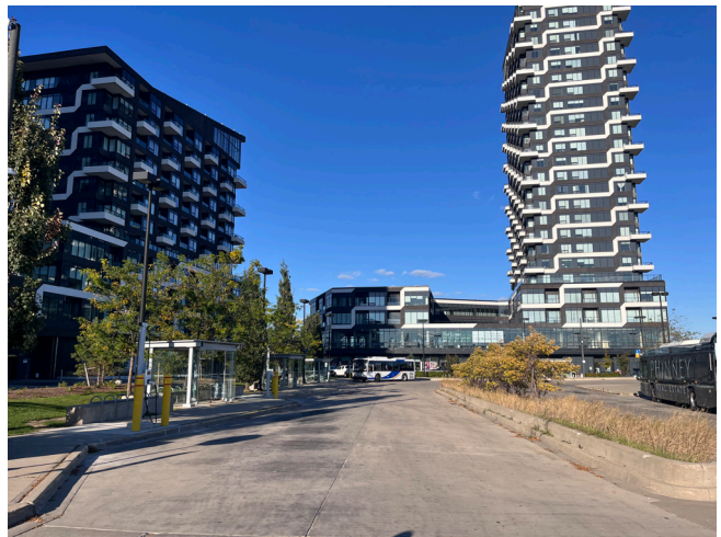
Figure 14. Uptown Core Terminal, which features bus shelters, seating, landscaping, e-charging ports, a staff rest facility, and bike repair equipment.
