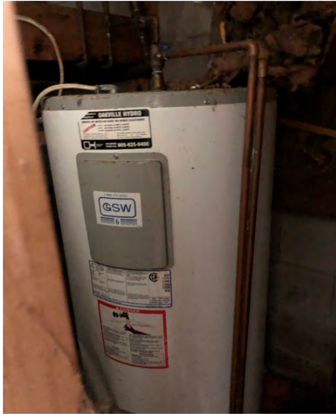
Photo 7: Interior of the Site Building
