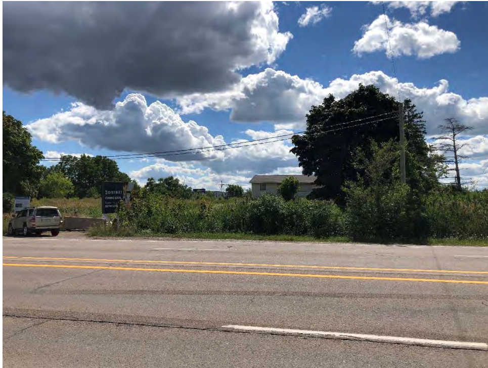
Photo 1: Frontage of 3064 Trafalgar Road, facing west.
