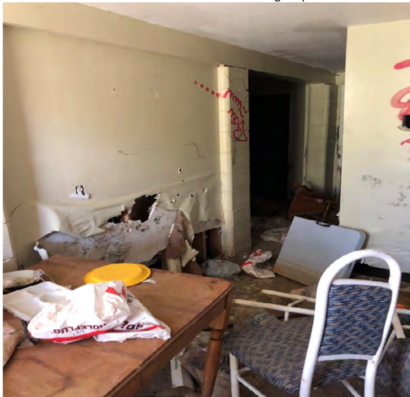
Photo 6: Interior of the Site Building
