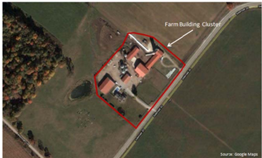
Farm Building Cluster
