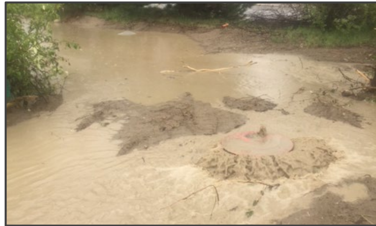
System Surcharge/ Basement Flooding
