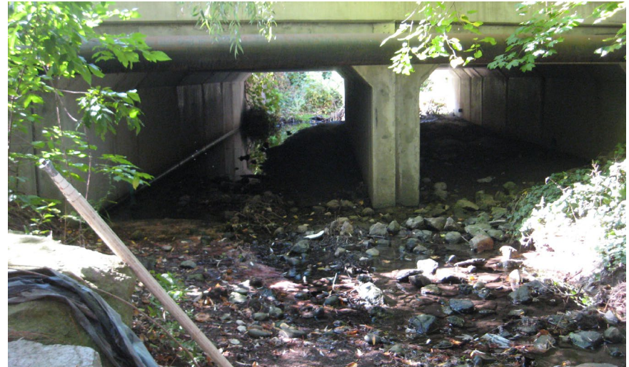
4: D/S Face of Chartwell Road Twin Conc. Box 3.0m x 1.9m, Station 176.7459
