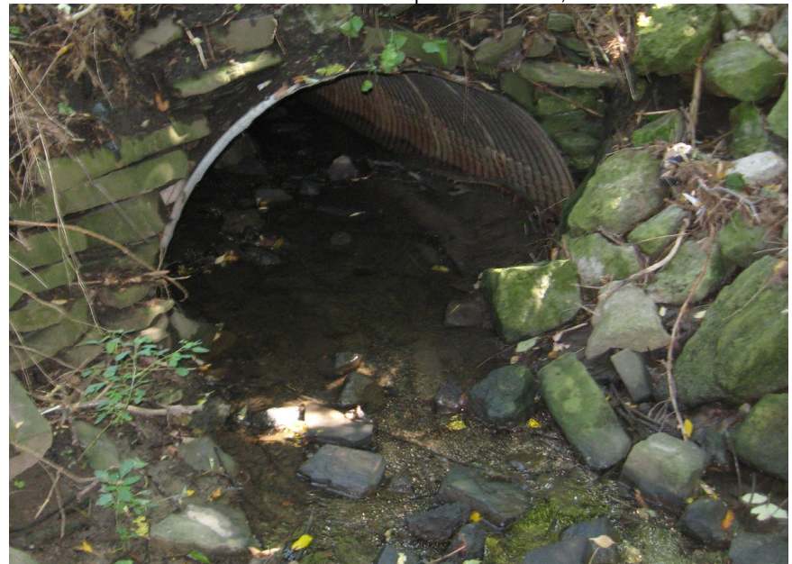
8: U/S Face Drummond Road CSP Arch 1.15m x 1.7m, Station 263.7177
