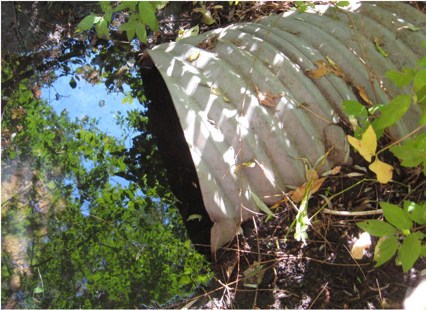
9: D/S Face Cumnock Crescent 600mm CSP, Station 409.8072
