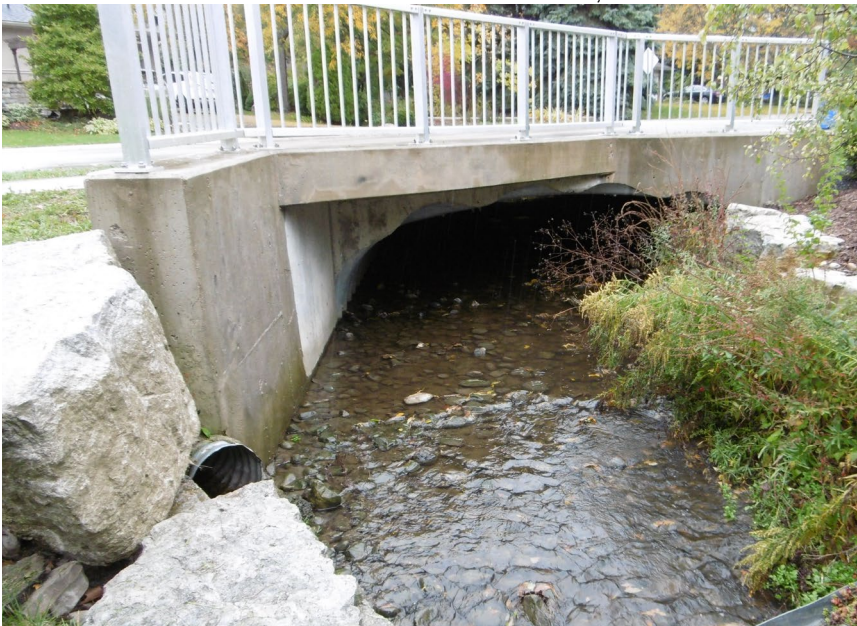
3: D/S Face of Wedgewood Drive 5.5m x 1.5m CSP Arch, Station 675.4334
