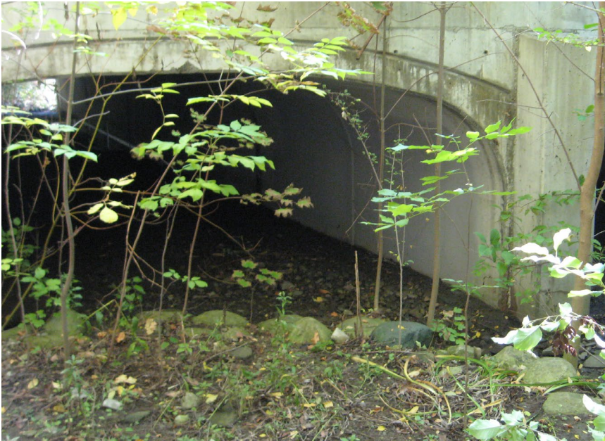
5: D/S Face Devon Road Twin Conspan Arch 4.3m x 2.0m, Station 1587.402
