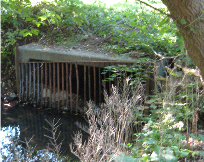
5: D/S Face Maple Avenue 3.0m x 1.2m Box Culvert, Station 2711.132
