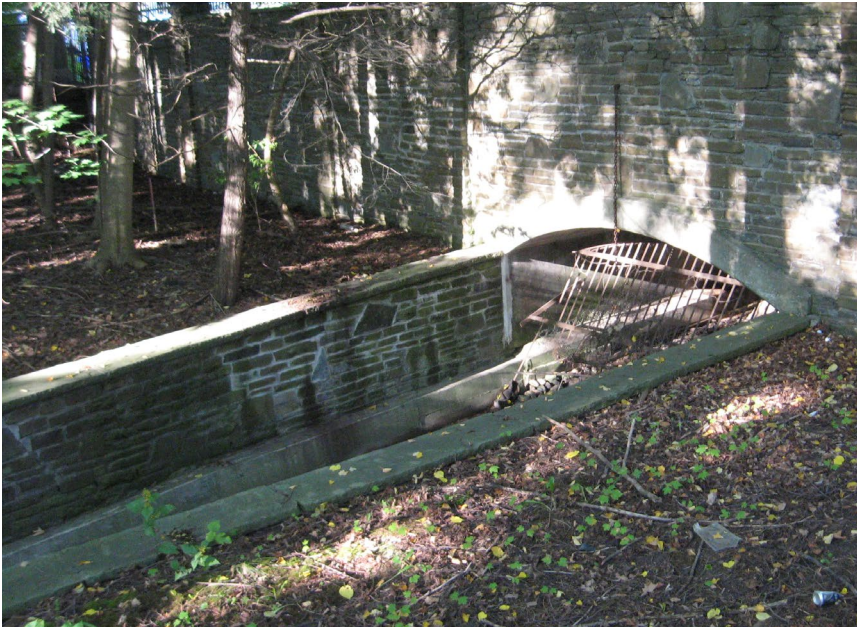
1: D/S Face Lakeshore Road 3.8m x 1.9m Conc Arch, Station 242.8122
