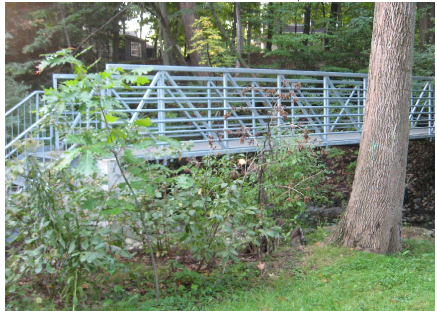
4: Bridge at Weaver Avenue Pedestrian Bridge 2.3m x 14.1m, Station 1480.446
