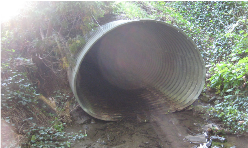
7: U/S Face Duncan Road culvert CMP Ellipse 2.45m x 1.8m, Station 1844.065
