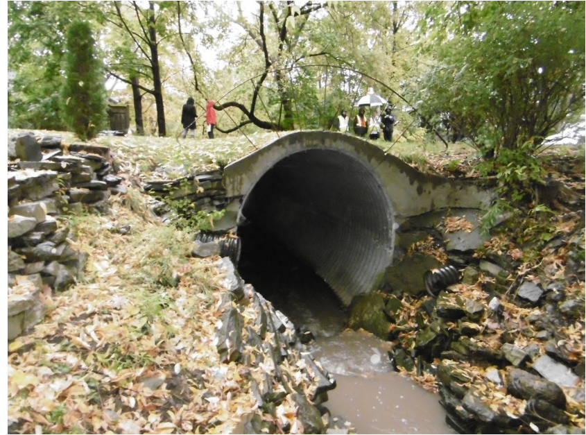
6: U/S Face of Amber Crescent CSP Ellipse 2.6m x 2.1m, Station 1711.164
