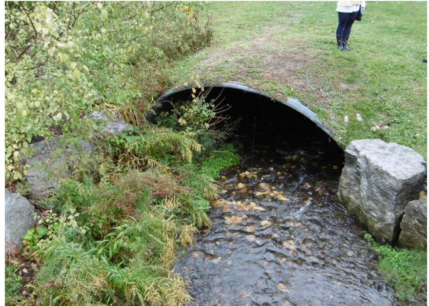
2: U/S Face of Warren Drive Park 4.2m x 1.5m CSP, Station 644.3186
