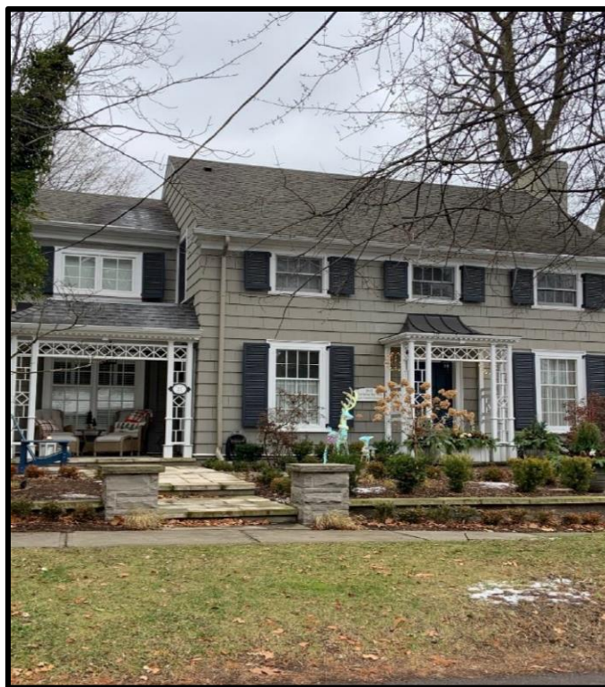
Figure 14: 27 Reynolds Street – Asphalt gable roof with shake cladding
