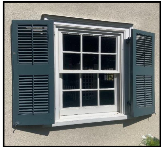
Figure 19: 308 William Street (left) – Wood windows with storm and operating louvered shutters Figure 20: 65 Navy Street (right) – Wood windows with thermal pane and operating louvered shutters
