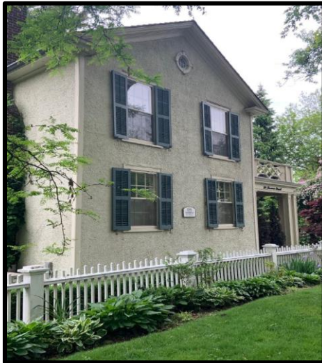
Figure 48: 29 Thomas Street (left) – Example of stucco cladding
