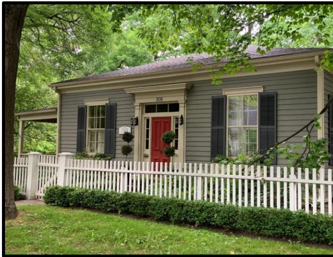
Figure 19: 308 William Street (left) – Wood windows with storm and operating louvered shutters Figure 20: 65 Navy Street (right) – Wood windows with thermal pane and operating louvered shutters
