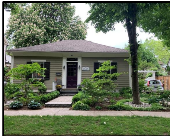
Figure 10: 329 William Street (left) – Cedar shake hip roof with stucco cladding Figure 11: 307 William Street (right) – Asphalt hip roof with horizontal wood cladding
