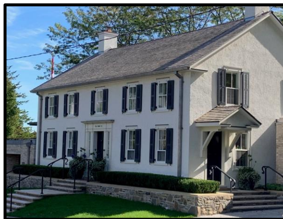
Figure 8: 212 Front Street (left) – Cedar shake hip roof with dormers and stucco cladding Figure 9: 176 Front Street (right) – Cedar shake gable roof with stucco cladding
