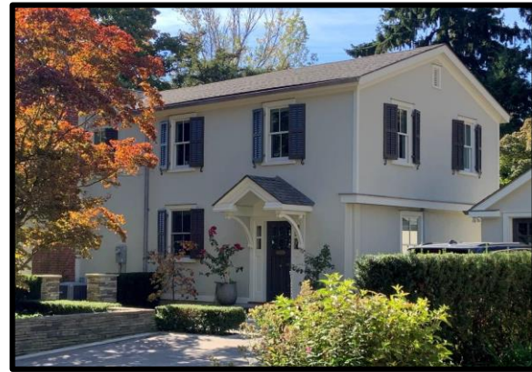
Figure 46: 53 Thomas Street (left) – Example of stucco cladding
