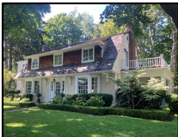
Figure 52: 309 King Street (left) – Example of stucco cladding with shake dormers
