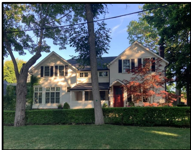
Figure 58: 273 William Street (left) – addition to west; height of addition matches; consistency in roof form and style of windows/doors and trim; complementary use of materials
