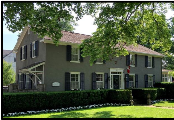
Figure 46: 53 Thomas Street (left) – Example of stucco cladding
