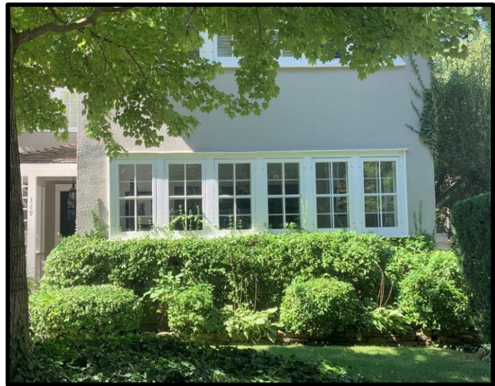
Figure 17: 24 Thomas Street (left) – Wood window with storm
