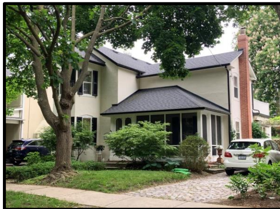
Figure 12: 65 Navy Street (left) – Asphalt gable roof on house and garage with stucco cladding Figure 13: 301 William Street (right) – Asphalt gable roof with stucco cladding
