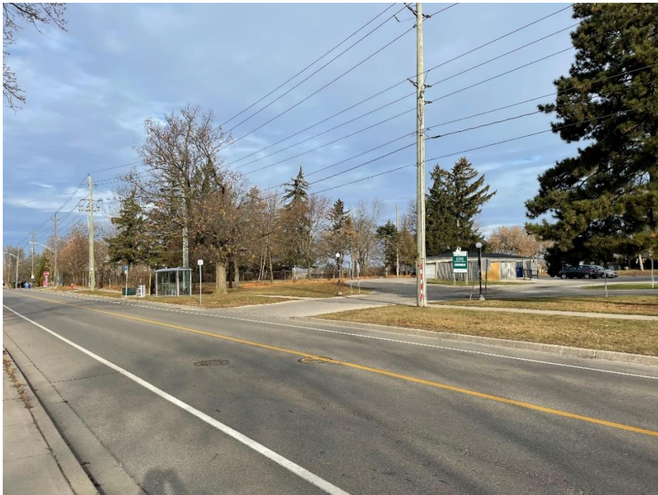
Image 11- Looking northeast across Sixth Line at the Castle Green Apartment driveway access and the Subject Lands
