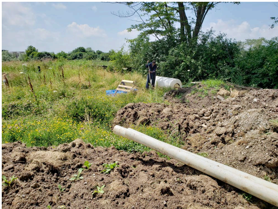
Photo 9: Southside of house, adjacent to septic tank and tile bed. Dumped piles of soil next to undisturbed area. Facing northwest. Grassed area subject to 5-metre interval test pit survey.
