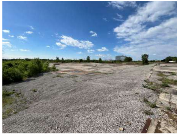
Photo 8: View of the south central portion of the Site. Photograph taken facing southwest.
