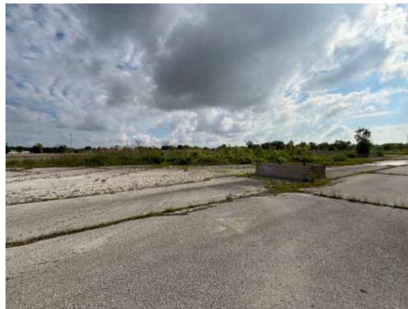
Photo 4: View of the south-central portion of the Site. Photograph taken facing southeast.
