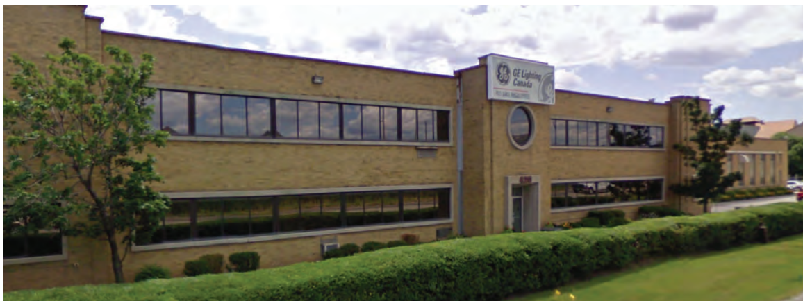
Figure 4. GE Lamp Plant Office Building. (Source: Google Street View)
