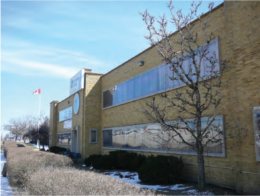
Figure 5. Office Building, looking East. (Source: ERA Architects)
