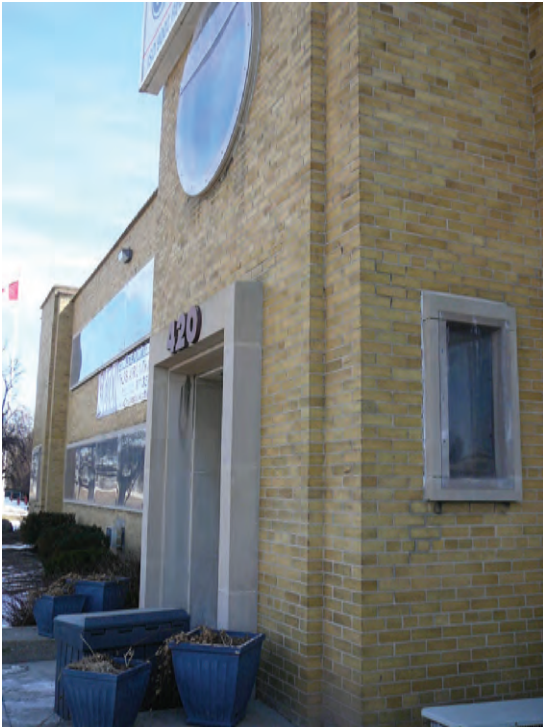
Figure 6. Office Building, entrance. (Source: ERA Architects)
