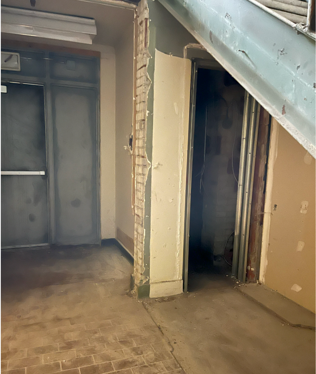
On the interior of the office building looking toward the main entrance (ERA, September 23, 2024).
