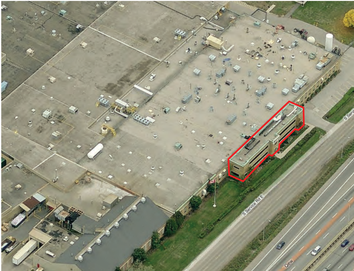
Figure 17. Office Building proposed for retention. (Source: Bing Maps)
