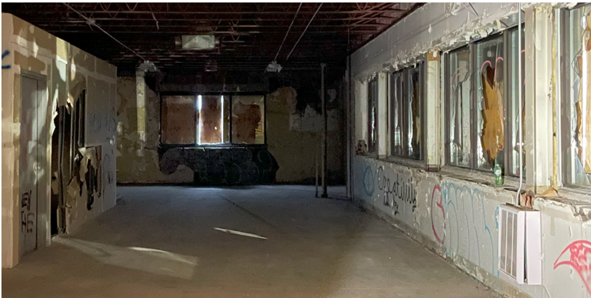
Standing in the east wing looking east toward the secondary staircase and beyond, where the building's original kitchen was located (ERA, September 23, 2024).
