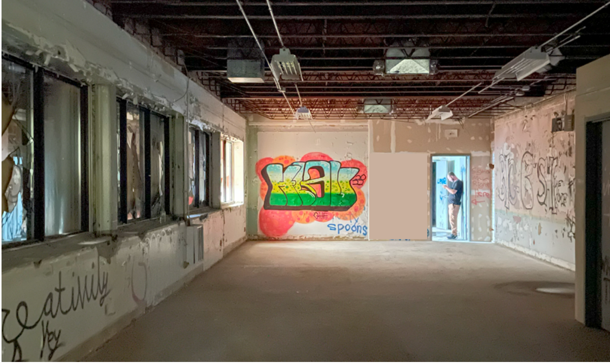
Standing in the east wing looking west toward the partition wall between the stairwell and the east wing (ERA, September 23, 2024).
