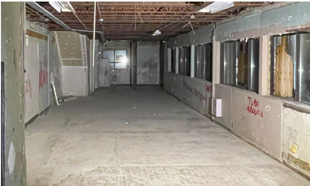
Looking toward the east wing on the first storey of the office building (ERA, September 23, 2024).
