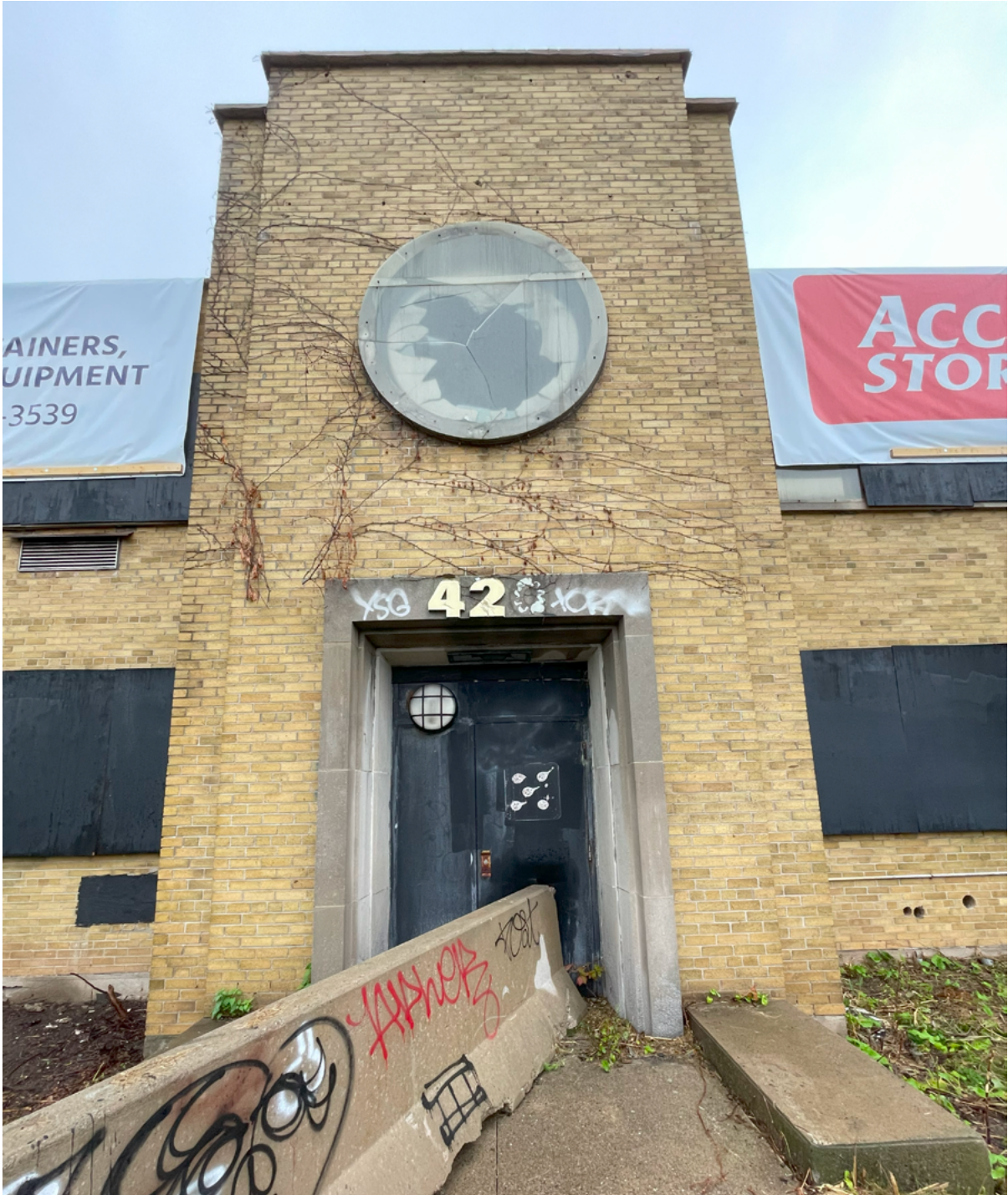
Looking toward the main entrance at the principal (northern) elevation of the office building (ERA, September 23, 2024).
