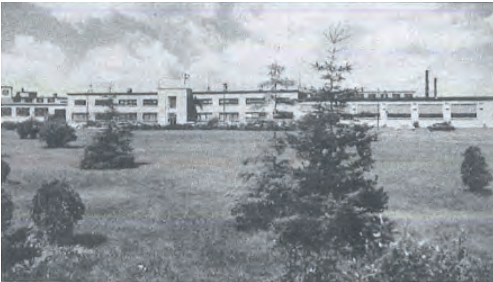
Figure 14. Original south elevation of the GE Lamp Plant, 1948. (Source: GE Lighting)
