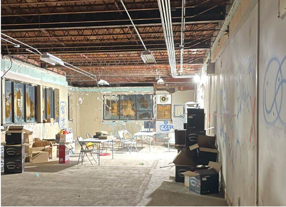
Looking toward the west wing on the first storey of the office building (ERA, September 23, 2024).
