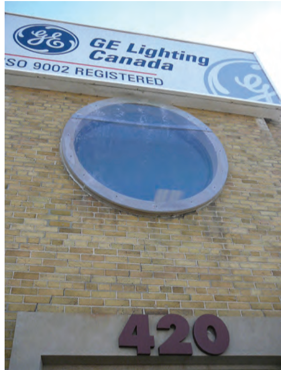
Figure 7. Office Building, second storey circular window. (Source: ERA Architects)
