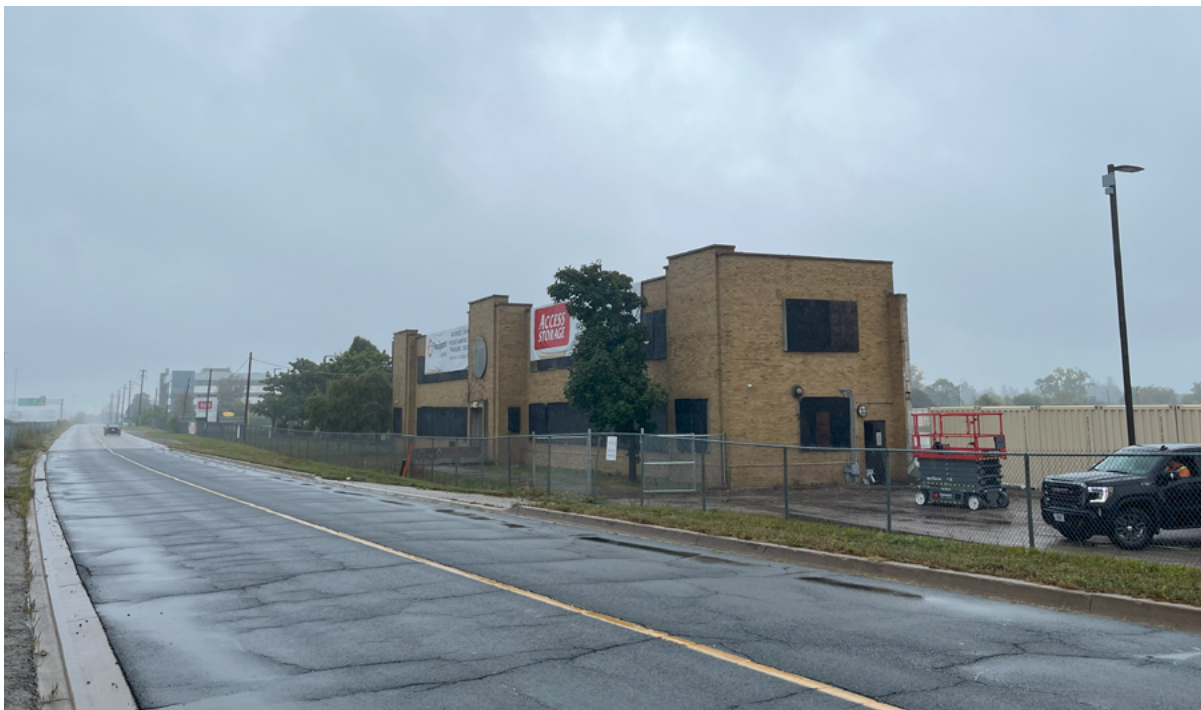
Looking northeast toward the principal (northern) elevation of the office building (ERA, September 23, 2024).
