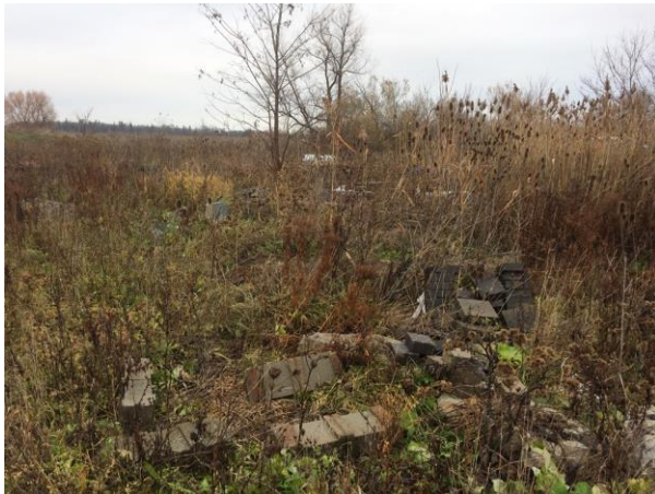
Plate 9. Scrublands and Building Debris (view north)
