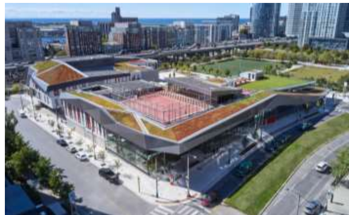
Canoe Landing Campus School, Toronto Source: ZAS Architects + Interiors
