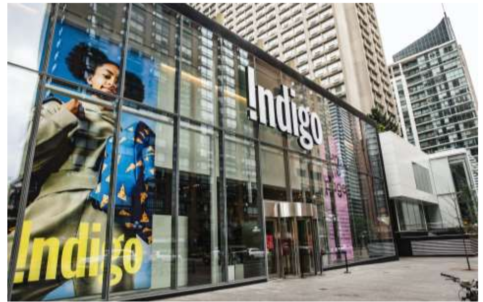
Manulife Centre, Toronto. Source: Manulife Centre
