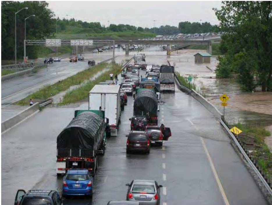
City of Hamilton - Red Hill Valley Parkway near Barton Street (July 26, 2009)
