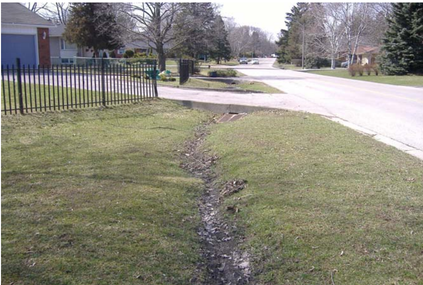
Photo 64: Looking north along west ditch of Woodhaven Park Drive.
