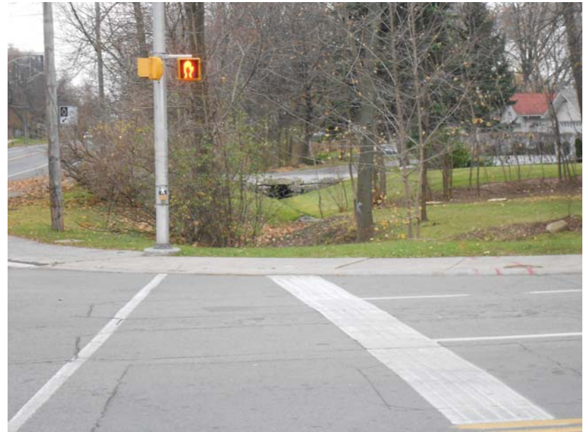
Photo 24: Looking west along Lakeshore Road across Third Line to open channel.
