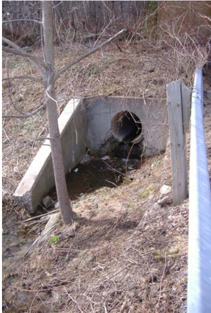
Photo 77: Storm sewer outfall adjacent to Lakeshore Road.
