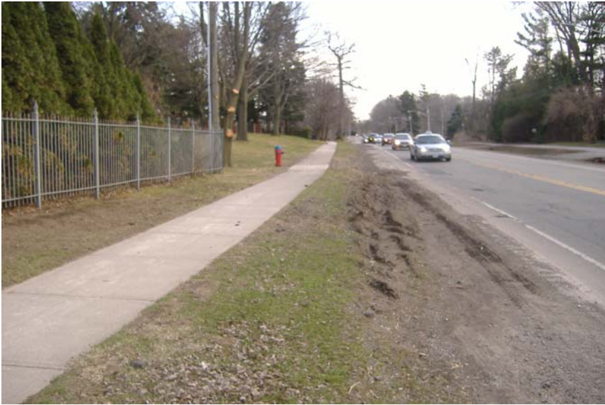
Photo 85: Looking west along south side of Lakeshore Road. Note lack of ditch.
