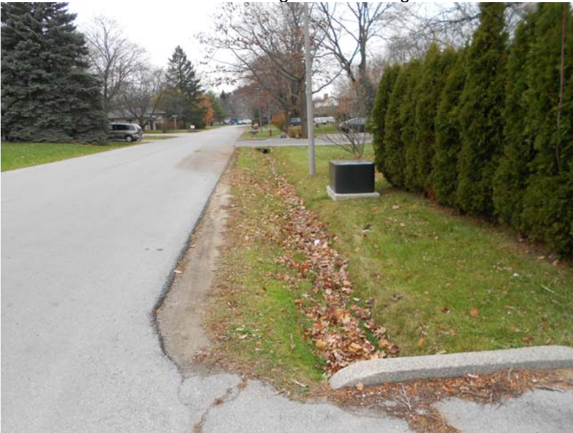
Photo 11: Looking upstream along east ditch of Westminster Drive.
