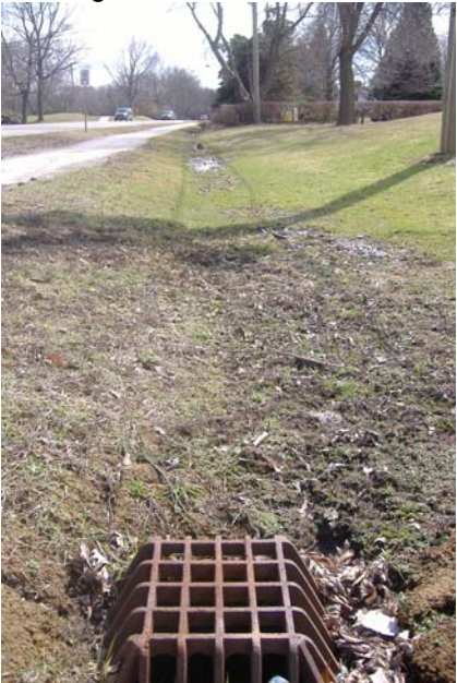
Photo 68: Looking west from catchbasin manhole along Lakeshore Road.
