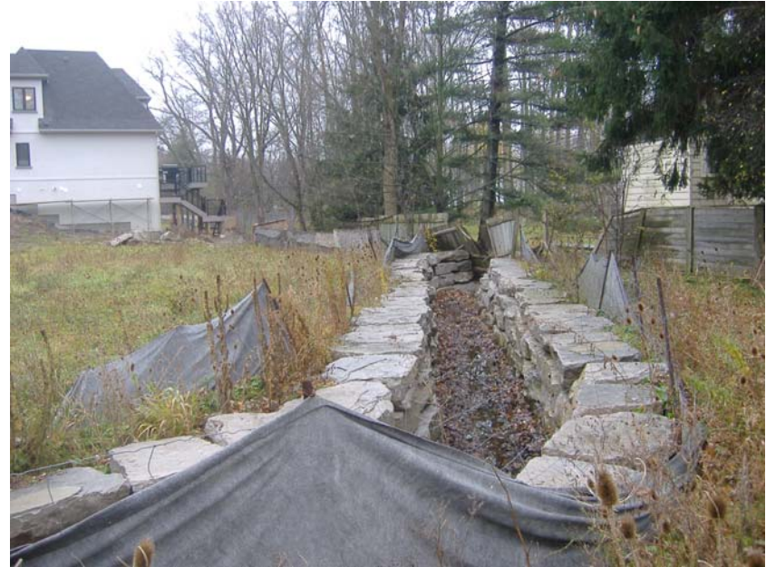
Photo 18: Looking downstream at recently constructed armour stone channel from Belvedere Drive.
