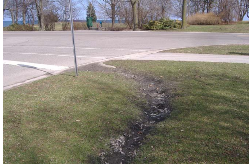
Photo 63: Curb cut at Lakeshore and Woodhaven Park Drive. Note sedimentation.
