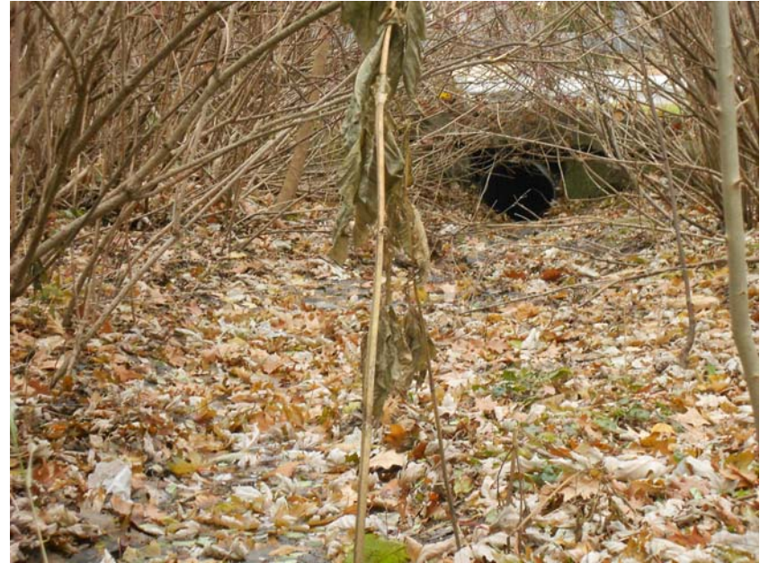
Photo 10: Looking upstream at culvert crossing.
