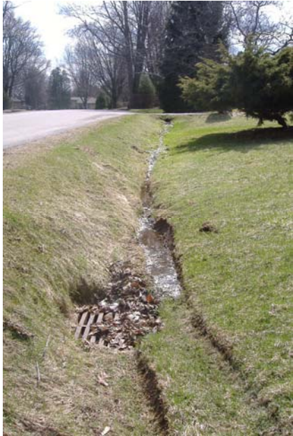
Photo 59: Looking west along Selgrove Crescent. Note tire tracks and significant erosion.
