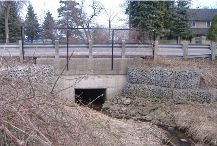
Photo 74: Upstream face of Lakeshore Road culvert.
