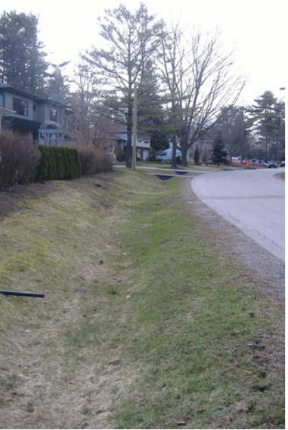
Photo 81: Looking along west ditch on Sandwell Drive.
