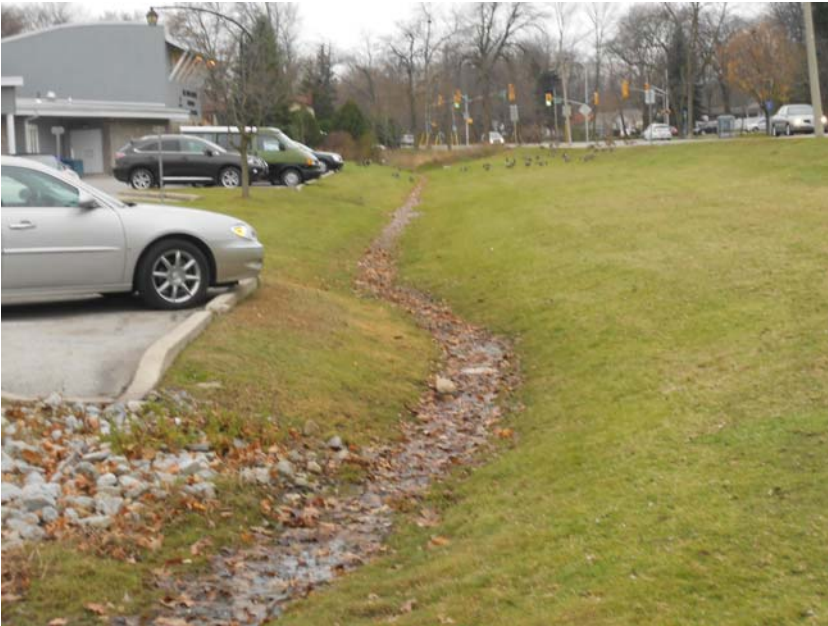
Photo 19: Looking upstream at open channel adjacent to Lakeshore Road. Note standing water.
