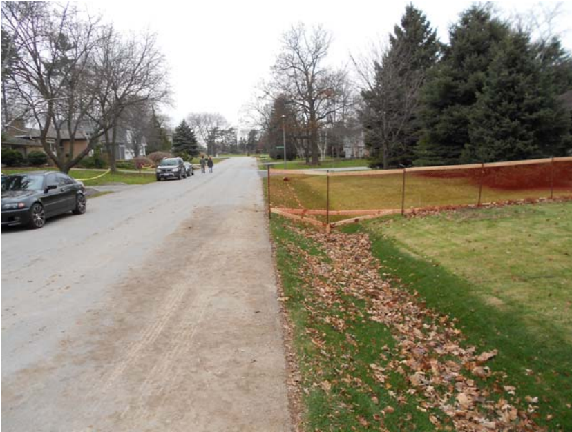
Photo 17: Looking upstream along east ditch of Westminster Drive.
