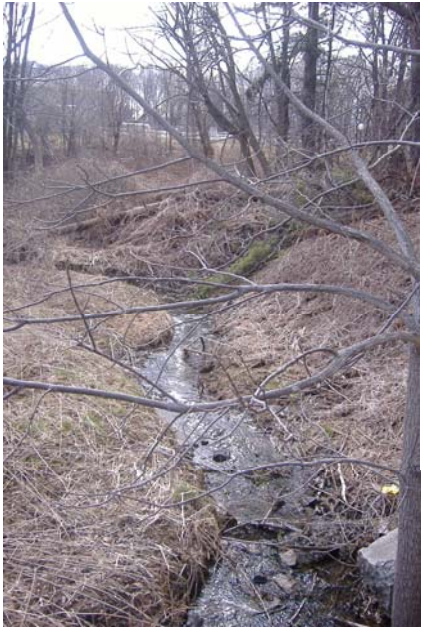
Photo 78: Looking upstream at open channel from Lakeshore Road.
