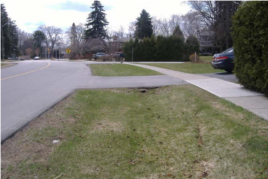
Photo 27: Looking west on north side of Hixon at Tracina. Note filled ditch/culvert.
