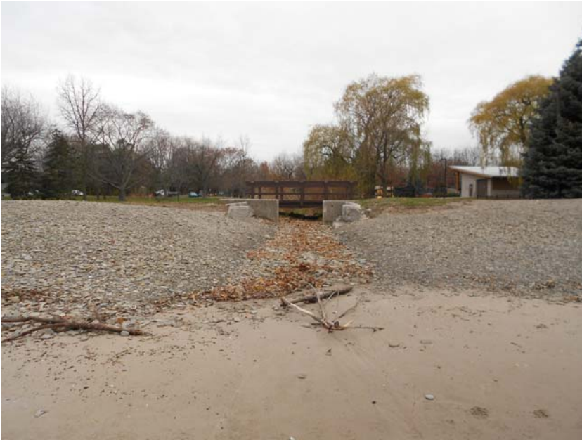
Photo 1: Looking upstream at channel and pedestrian bridge from Lake Ontario.
