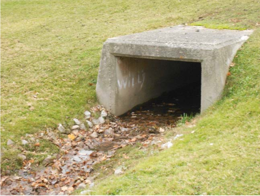
Photo 25: Looking at downstream face of culvert crossing of Lakeshore Road.
