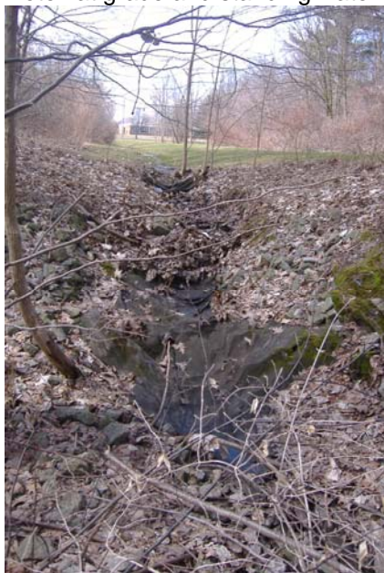
Photo 48: Looking upstream at ditch outfall. Note exposed erosion blanket and channel erosion.
