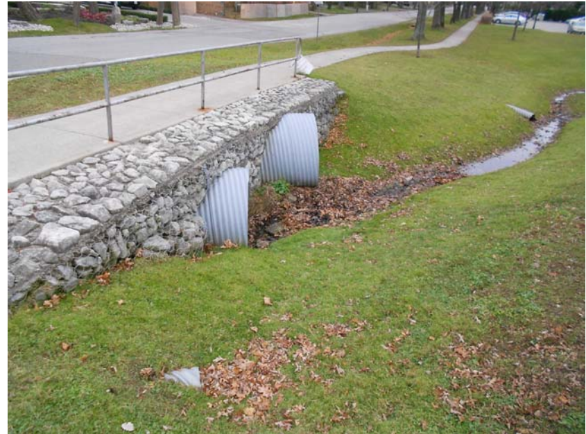
Photo 20: Looking at upstream face of culvert crossing of Old Lakeshore Road.
