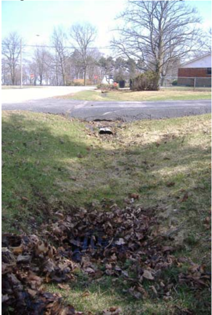
Photo 60: Looking south along west ditch of Woodhaven Park Drive. Note obstructed catchbasin and crushed culvert.
