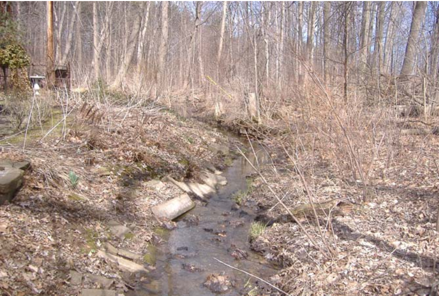
Photo 54: Looking downstream at open channel behind Hixon Street. Note bank erosion.
