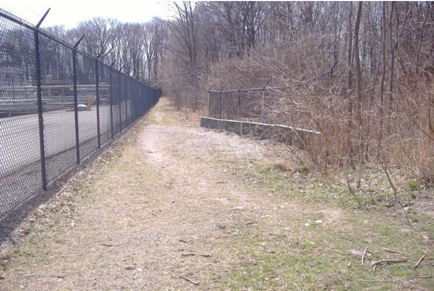
Photo 50: Looking downstream at headwall for culvert, and fence for WWTP site.
