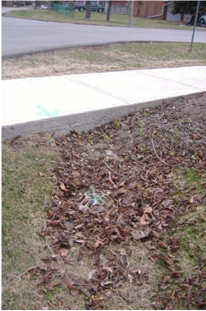
Photo 30: Beehive CB at north-west corner of Tracina/Hixon. Note debris blockage.
