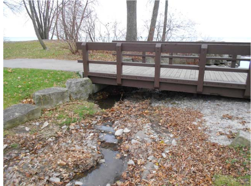
Photo 6: Looking downstream at pedestrian bridge.
