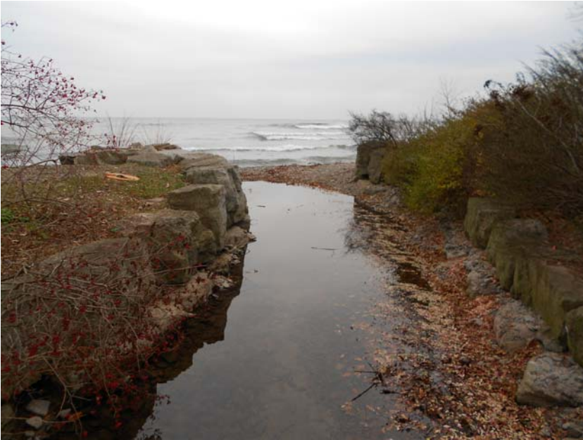
Photo 5: Looking downstream to Lake Ontario from pedestrian bridge. Note standing water.
