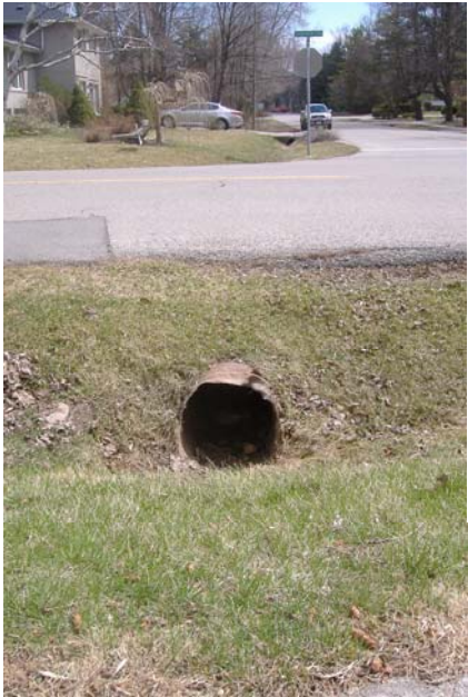
Photo 42: Upstream face of Sedgewick Crescent culvert.
