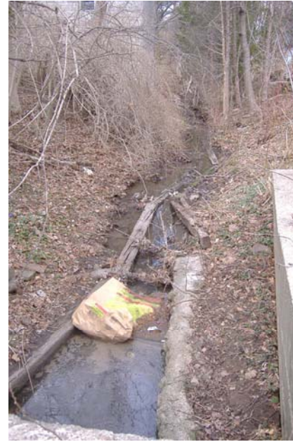
Photo 31: Looking downstream at storm sewer outfall at Willowdown Road. Note debris and minor erosion.
