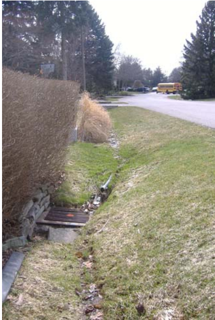
Photo 51: Looking west along Hixon Street at catchbasin manhole.
