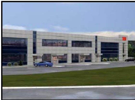
Office / Industrial Building Airport Rd & Mayfield Rd, Caledon 43,128 sq.ft
